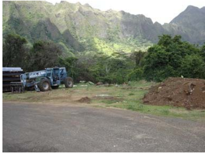
Figure 4. Proposed Verizon Hawaiian Memorial cellular site at Kōʻolau Golf Course maintenance facility, looking northwest. Photograph courtesy of Bureau Veritas.
