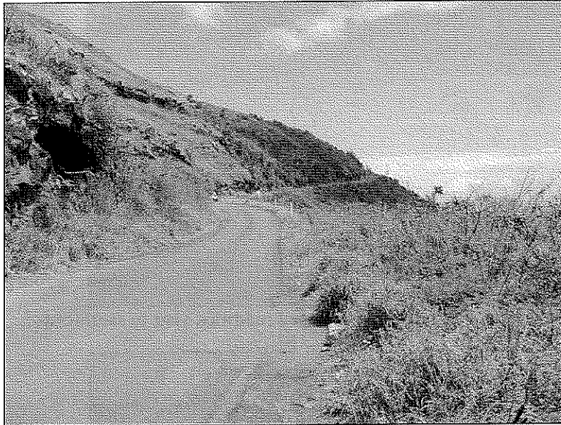
Photo 3: Overall view of beginning of the project area, view to the northeast.
