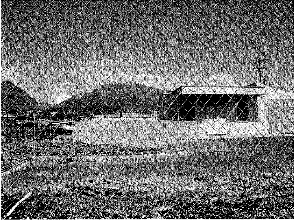
Photo 15. Wailuku WWPS facilities.
