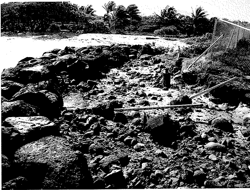
Figure 5. Damage at East End of the WWRF Revetment
