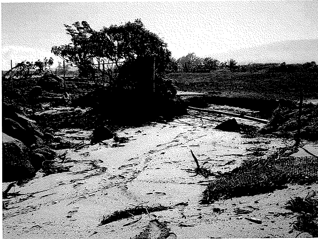
Figure 6. Damage at West End of the WWRF Revetment
