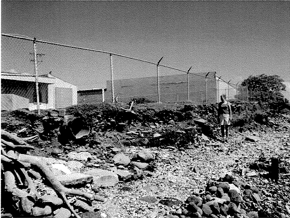
Photo 13. Large escarpment fronting the WWPS property (fence).
