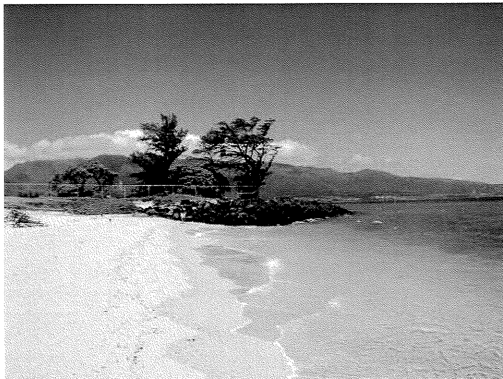
Figure 3. Looking West towards the Wailuku-Kahului WWRF revetment.
