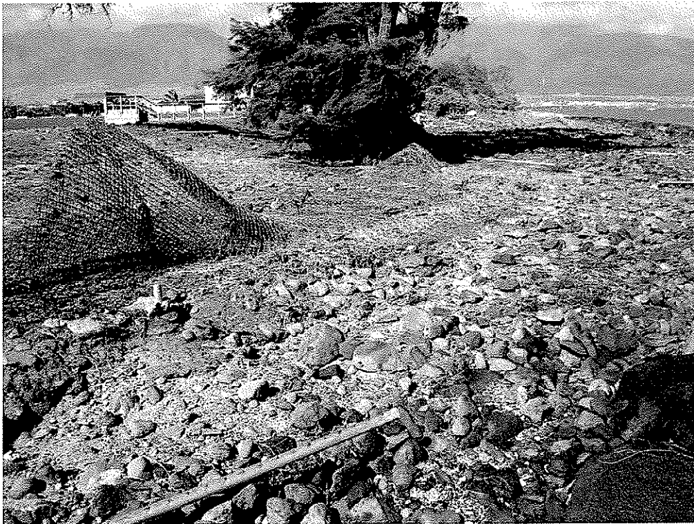
Figure 4. Looking West Along the WWRF Revetment
