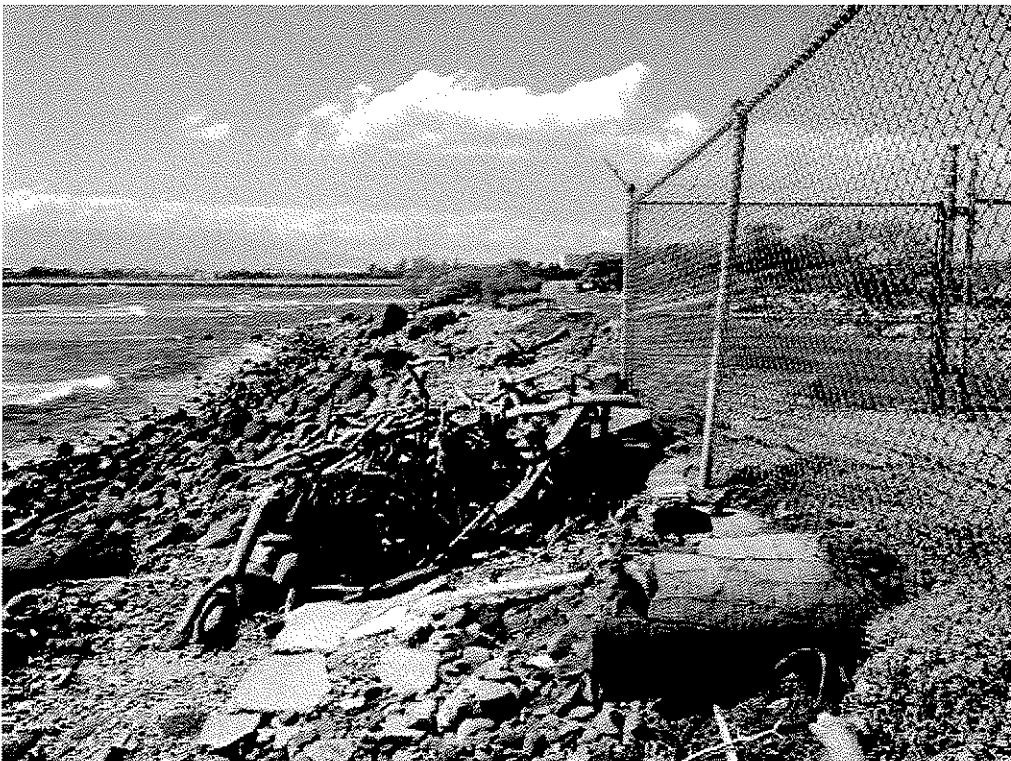
Photo 14. Looking Southeast along WWPS property line towards Kahului Harbor.
