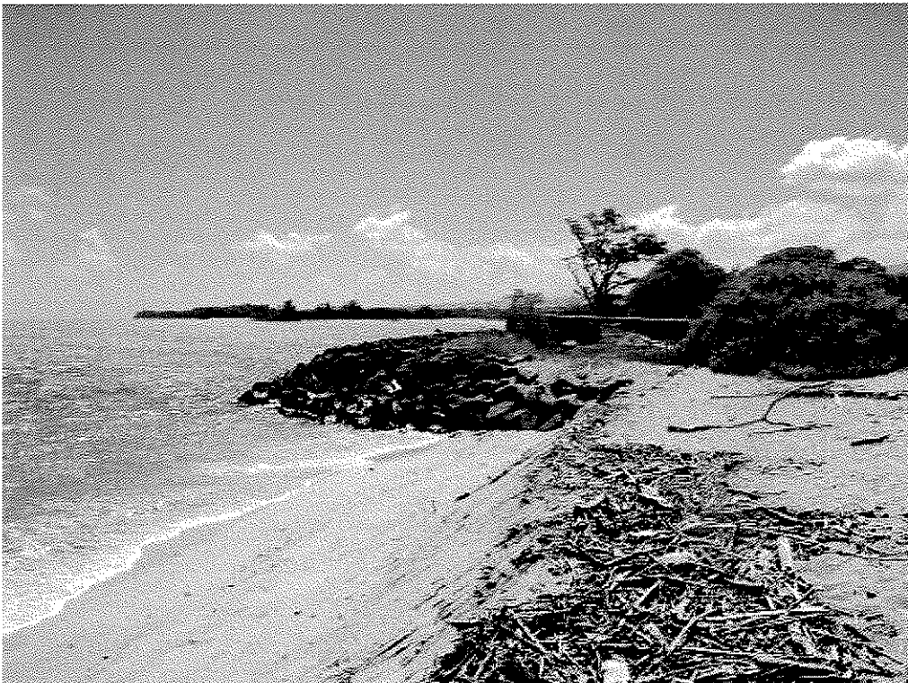
Photo 8. Looking East towards the revetment.
