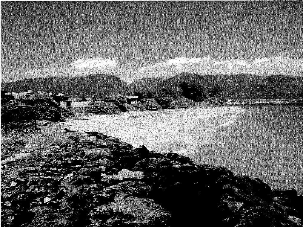
Photo 6. Looking West from the crest of the revetment towards Kahului Harbor.
