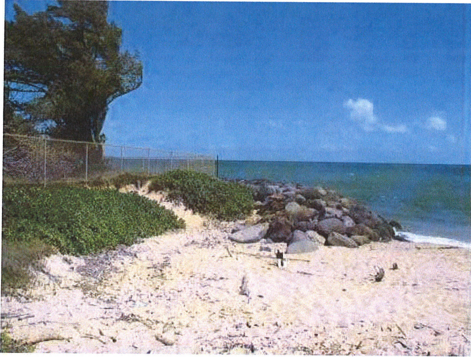
East Flank of Existing Revetment
