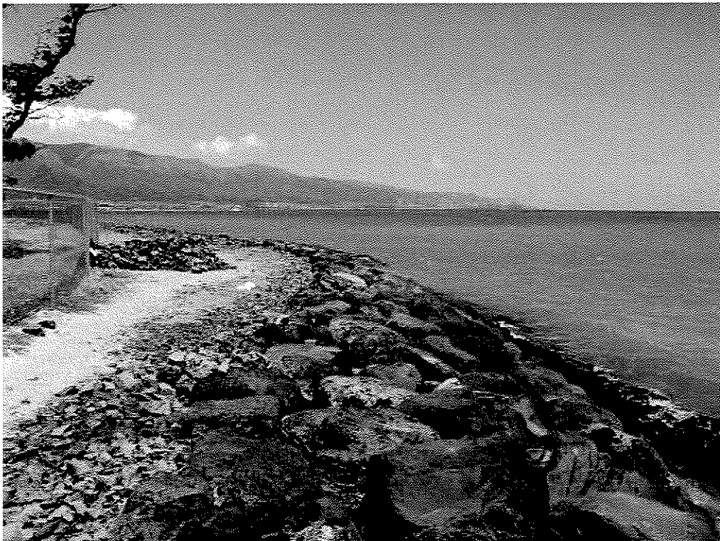
Photo 4. Looking West from the crest of the revetment towards Kahului Harbor.
