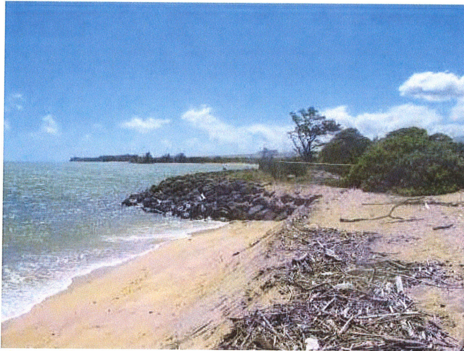
West Flank of Existing Revetment
