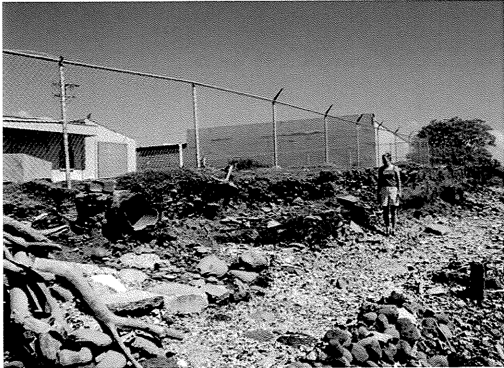
Figure 6. Large escarpment fronting the WWPS property (fence).
