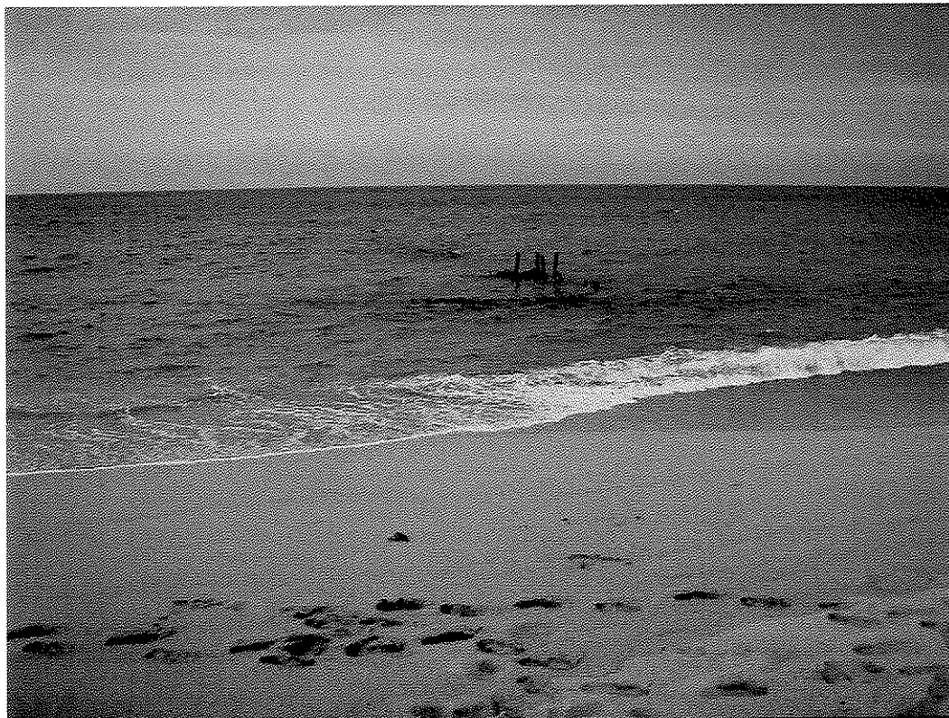
Figure 16. Outfall West of Revetment – 2007 (Rocks Buried and Beach Accretion)
