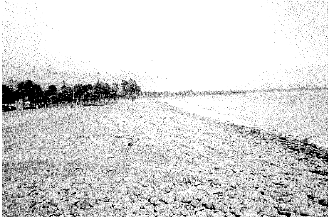
Figure 26. Picture of a cobble nourishment project, City of Ventura in Southern California.
