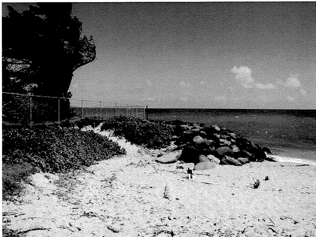
Figure 2. East flank of the revetment fronting the Wailuku-Kahului WWRF.
