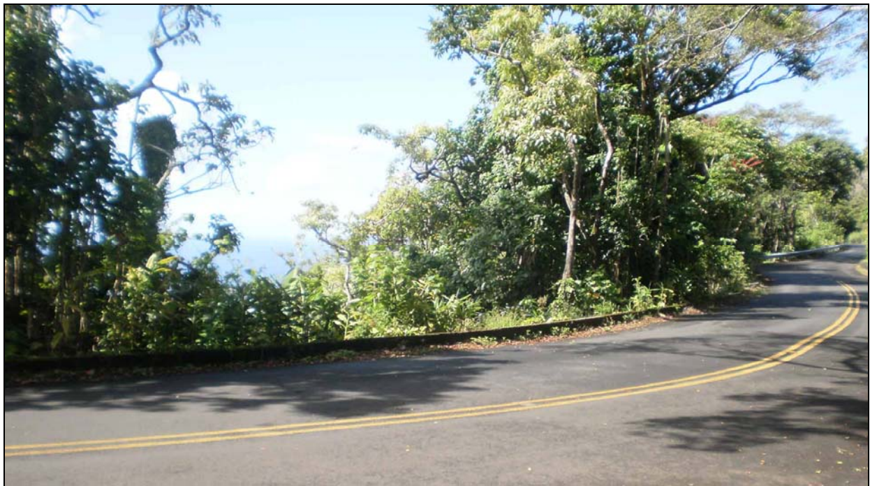
Figure 13. Photograph showing the low curb along the southeastern (Makiki Valley) side of Tantalus Drive, view to south
