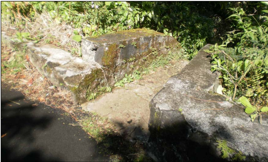
Figure 17. Photograph of the culvert showing the basalt and concrete construction of the sidewalls and the concrete floor, view to southwest.
