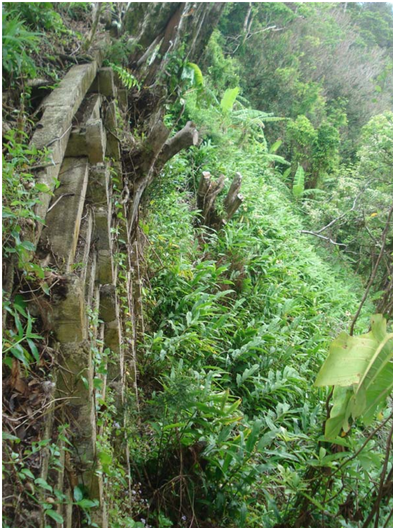
Photo 5. Crib wall structure supporting roadway
