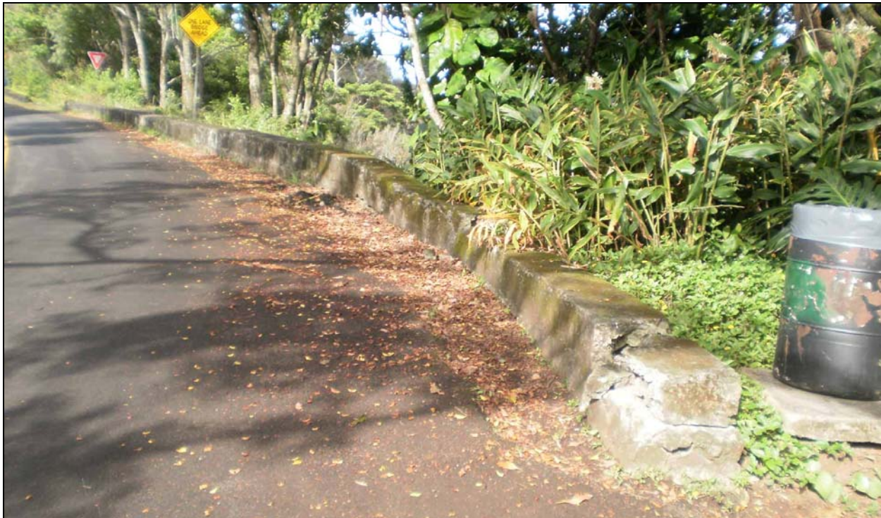
Figure 9. Photograph showing the low basalt and concrete guard wall along the northwestern (Pauoa Valley) side of Tantalus Drive, view to southwest
