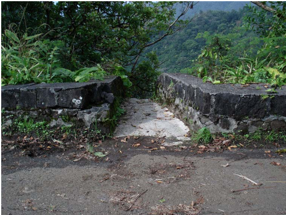
Photo 7. Spillway directs stormwater flow toward Pauoa Valley
