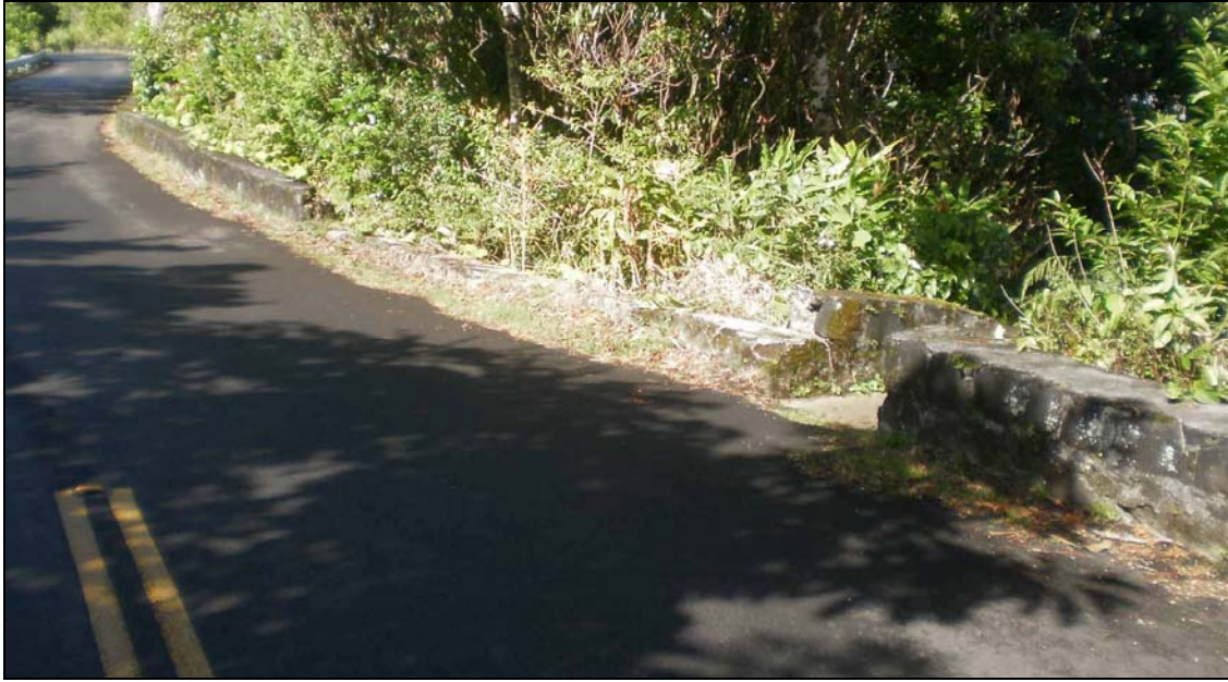
Figure 16. Photograph showing the culvert at the southern end of the low basalt and concrete guard wall along the southwestern (Pauoa Valley) side of Tantalus Drive, view to west. Note that the guard wall continues south of the project area along the ‘Hogsback.’
