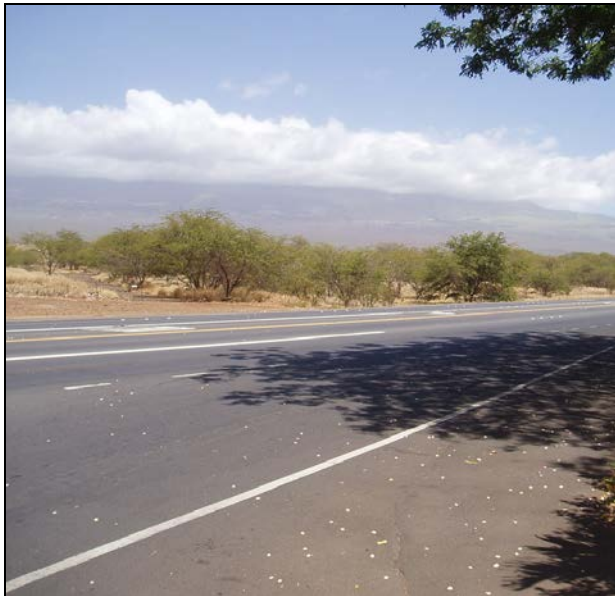
Figure 4-1114 (3) View From Pi'ilani Highway, Looking South
