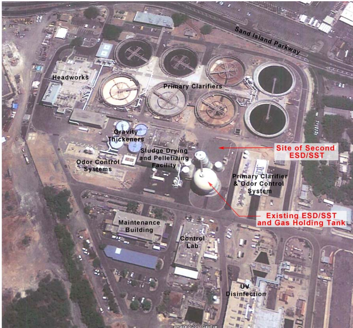
Figure 2-1, Aerial View of Sand Island WWTP
