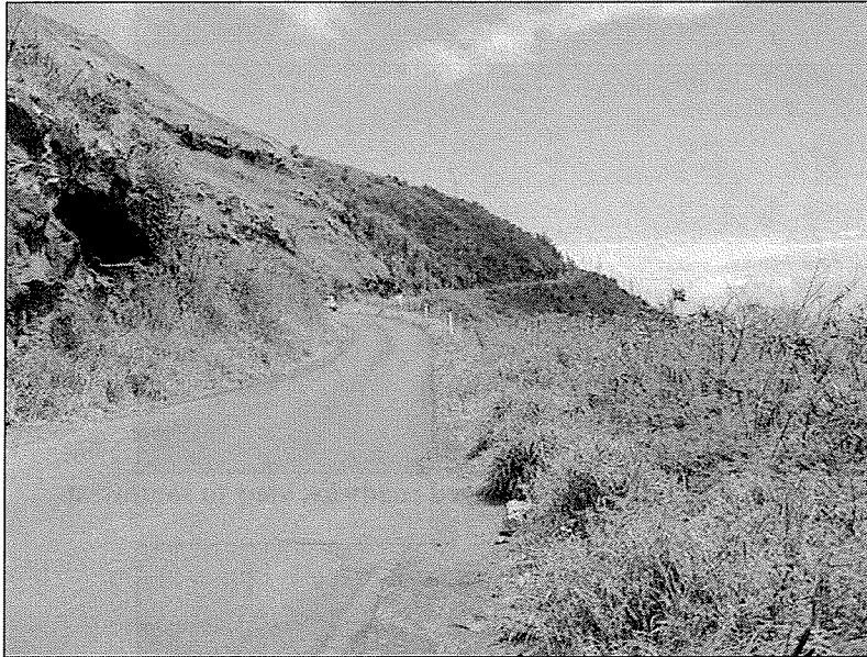
Photo 3: Overall view of beginning of the project area, view to the northeast.
