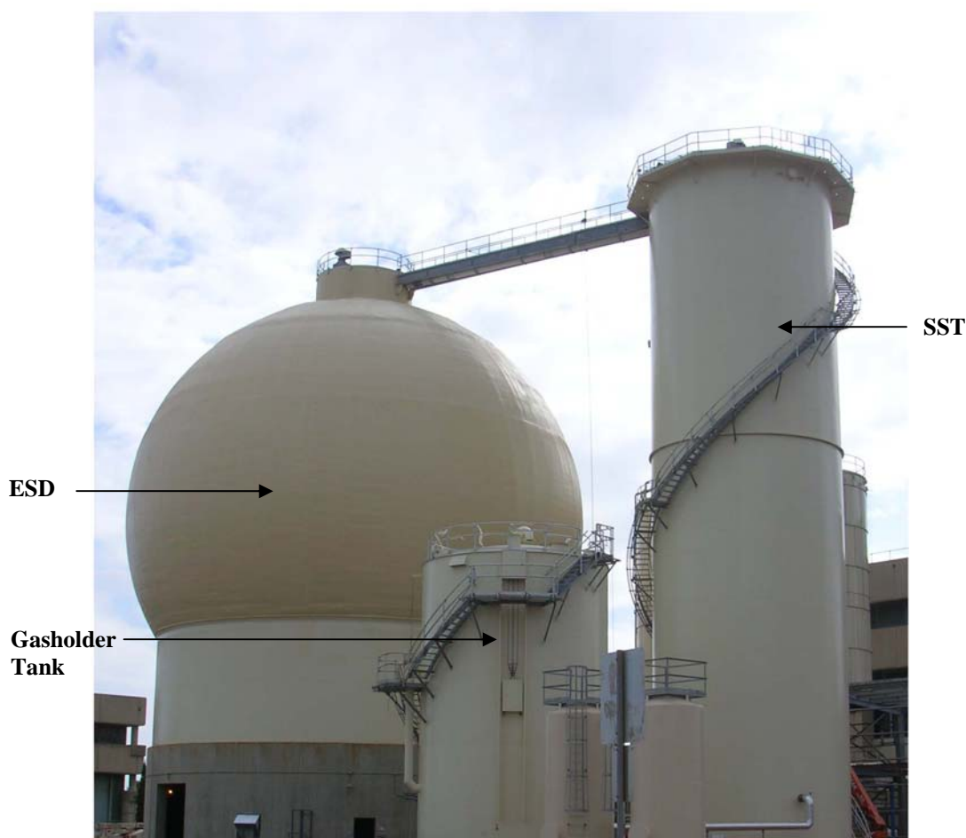
Figure 2-4, Photo of Existing ESD/SST and Gasholder Tank, Sand Island WWTP (Source: CB&I)
