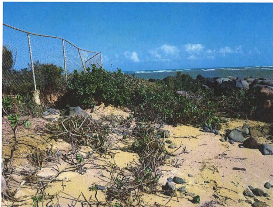
Photo No. 2: Erosion from Behind the East Flank, Which Undermined the Chain Link Fence Footings
