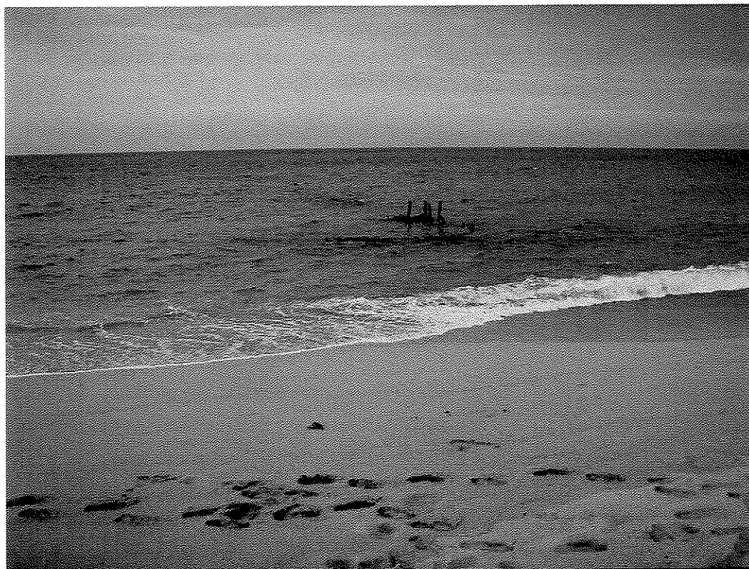
Figure 16. Outfall West of Revetment – 2007 (Rocks Buried and Beach Accretion)
