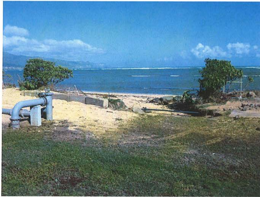
Photo No. 1: Scouring at West End of Revetment (pictured on the right)
