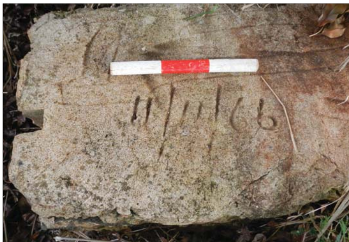
Figure 23: Detail photograph of the “11/11/66” date inscription on a site 50-30-08-2160, Ditch 1 sluice gate fitting, looking down. Note the grooves at the left of the frame for the sluice gate boards. Figure 22 depicts an expanded view of this sluice gate fitting. The scale is in decimeters.
