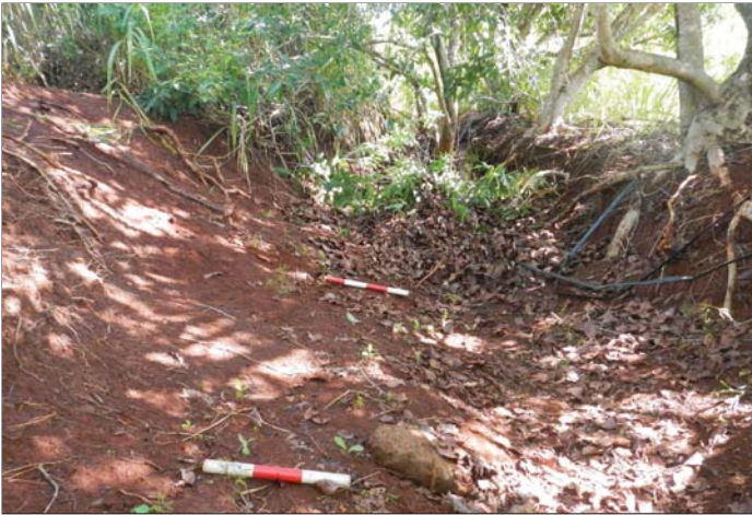
Figure 25: Photograph of the canal of site 50-30-80-2160, Ditch 2, looking east. Note the plastic irrigation pipe lying on the ground surface and extending from the walls of the linear mounds.
