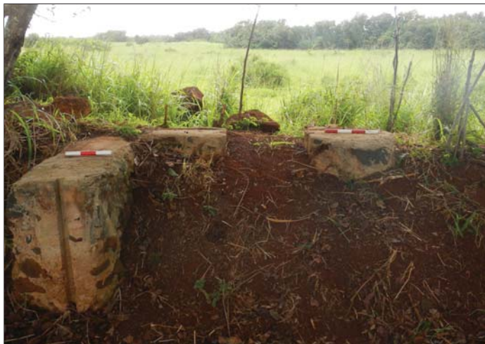
Figure 22: Detail photograph of the 1966 notched sluice gate fittings in Ditch 1 of site 50-30-08-2160, looking south. Note that the left scale bar marks the inscribed date (fig. 23). The scale is in decimeters.
