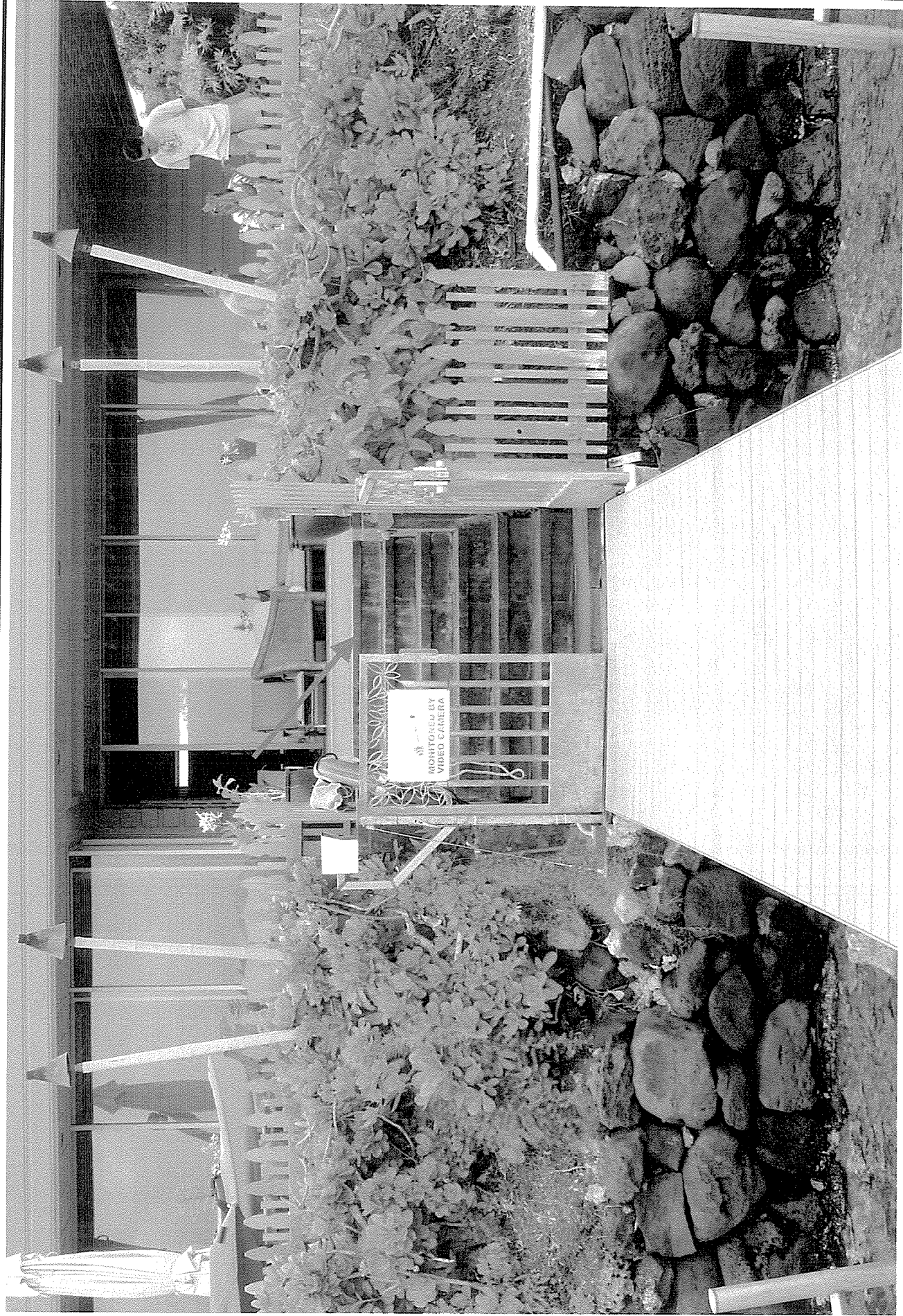
Picture taken from the pier on the shoreline looking towards the rear of the dwelling. The red arrow shows the existing grade of the backyard approximately 8-feet above the base of the seawall. The eroded condition of the rear slope of the property between the top of the crumbling seawall and the existing grade is visible. Picture 1
