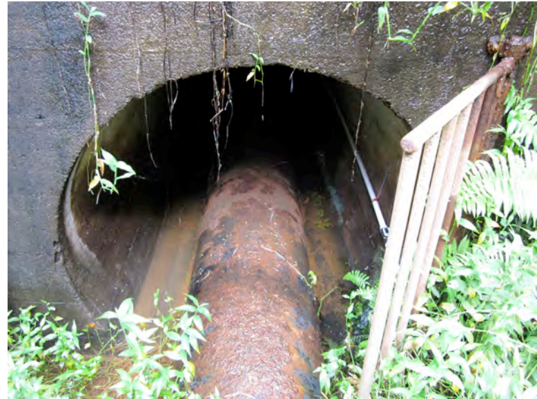
Photo 6: Outlet pipe emerging from base of dam at Nuuanu Reservoir #4.
