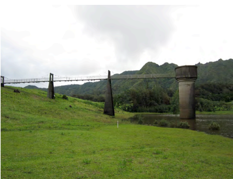
Photo 3: Side view of suspended bridge and intake tower.
