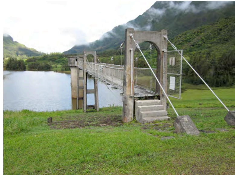
Photo 2: Suspended bridge leading to outlet works tower at Nuuanu Reservoir #4.
