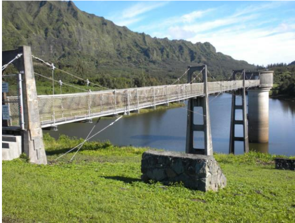
Figure 3-9: Reservoir Intake Tower
