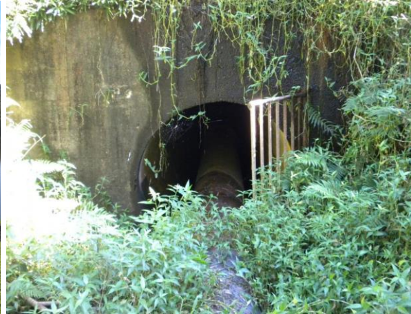
Figure 3-10: Reservoir Outlet Tunnel
