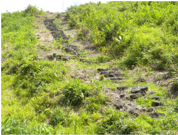
Figure 3-11: Access steps, Dam Embankment.
