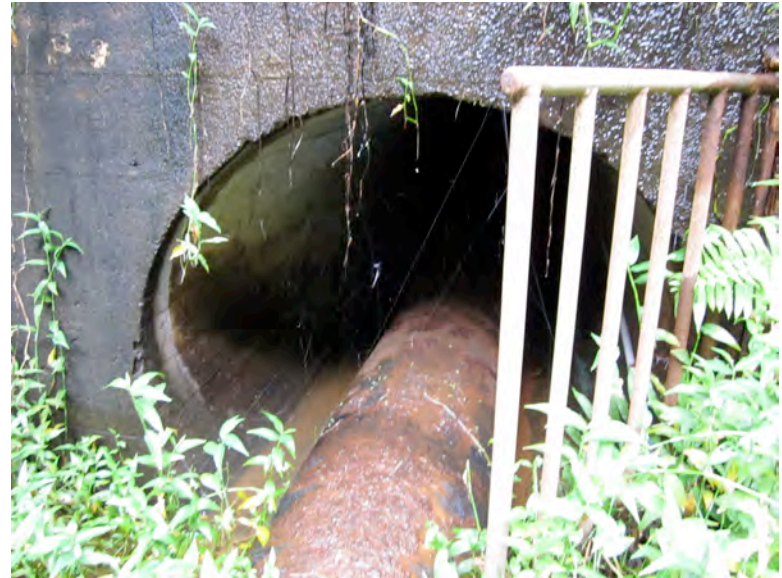
Photo 10: Steel outlet pipe emerges from Nuuanu Reservoir #4 dam.
