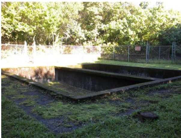
Figure 3-13: Sand Filter Pits (no longer used).
