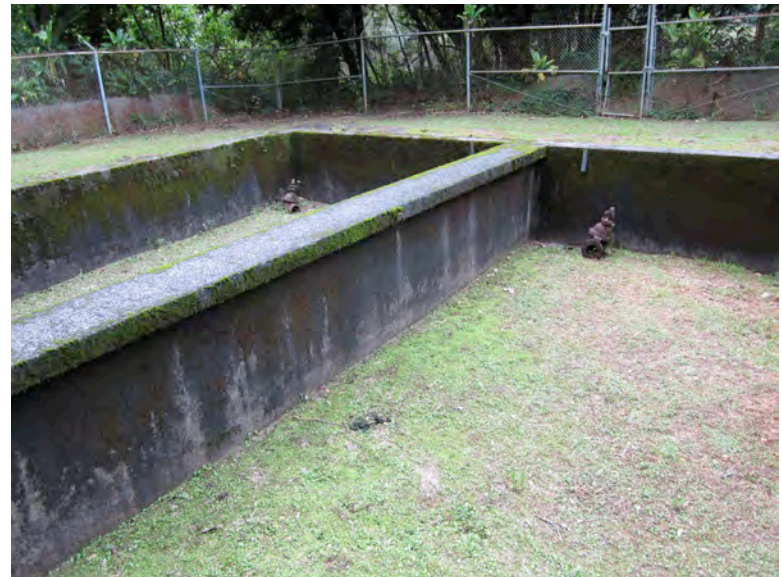
Photo 12: Close up of historic sand filter pits.
