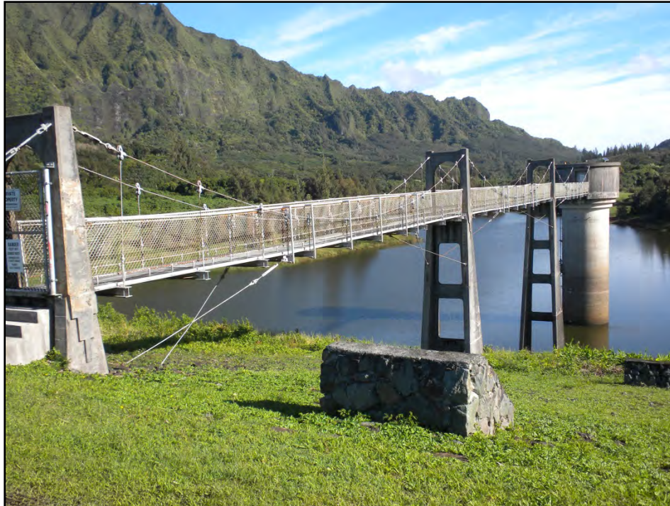
Figure 41. Intake tower and tower footbridge
