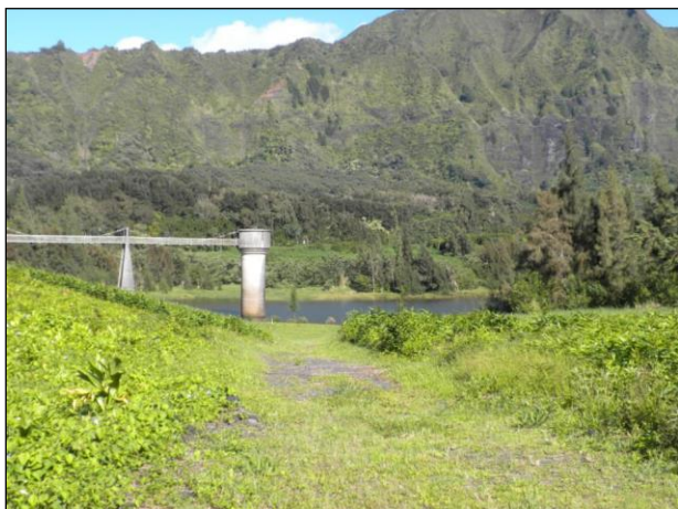
Figure 2-7: Spillway in Reservoir Basin.
