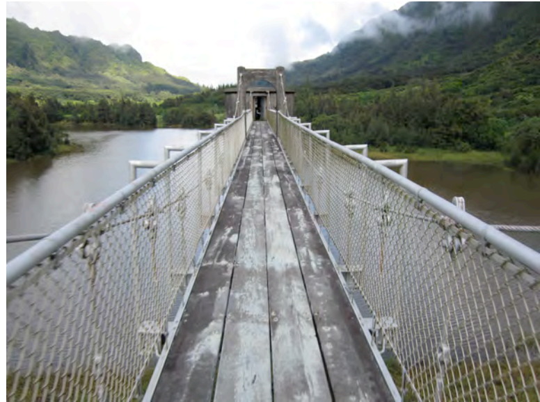
Photo 2: Suspended bridge leading to intake tower at Nuuanu Reservoir #4.
