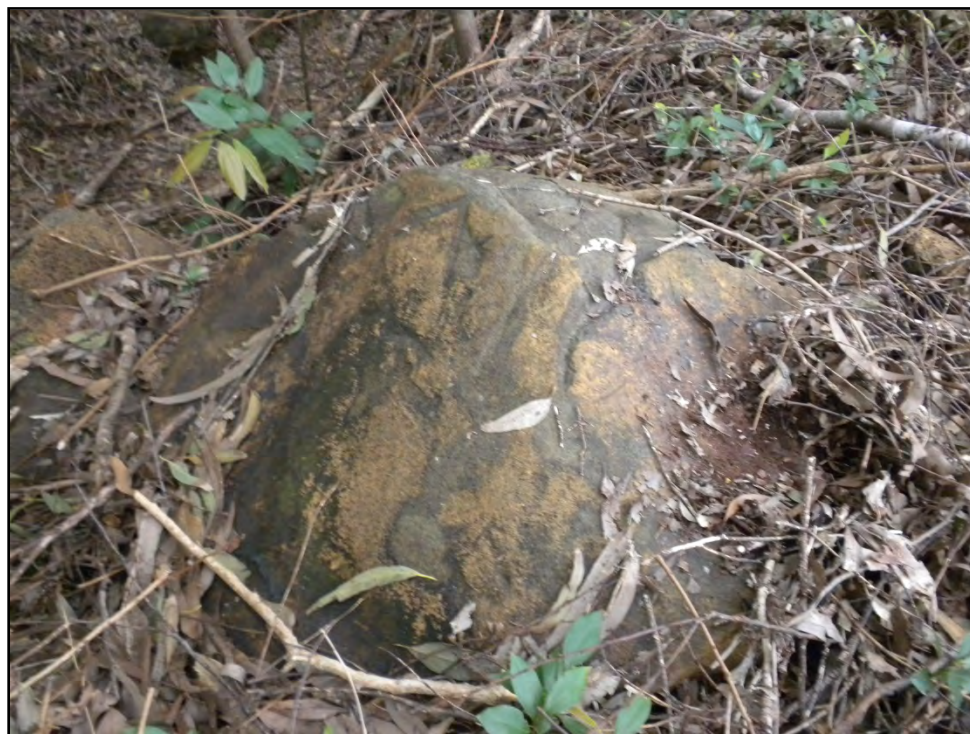
Figure 39. Dozer scarring on a boulder near the ditch
