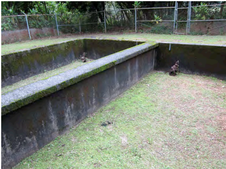
Photo 11: Close-up of sand filter construction.
