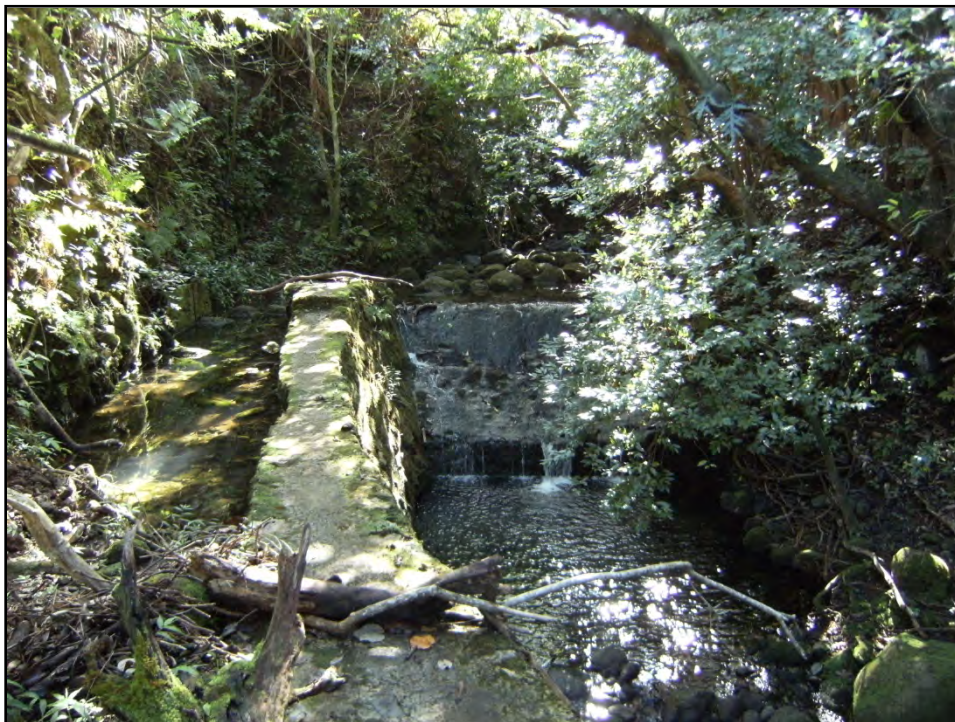
Figure 56. Concrete and rock wall/dam alongside a stream
