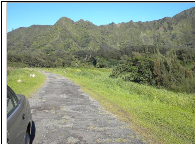
Figure 2-5: Access Road on Dam Crest.
