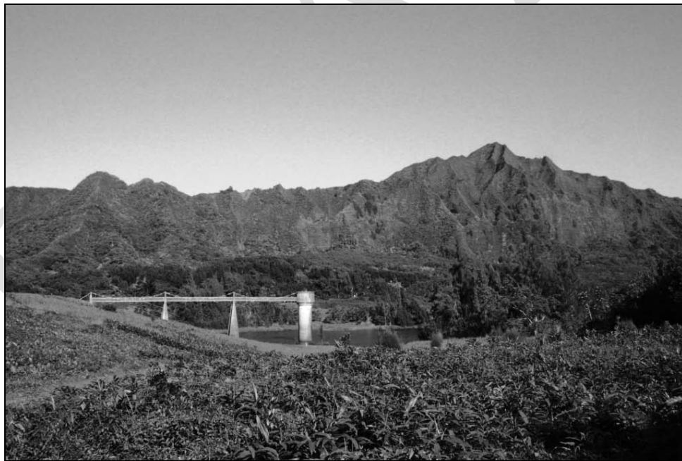
Figure 42. Nu'uanu Reservoir No. 4, with spillway in the foreground (CSH January 9, 2011)
