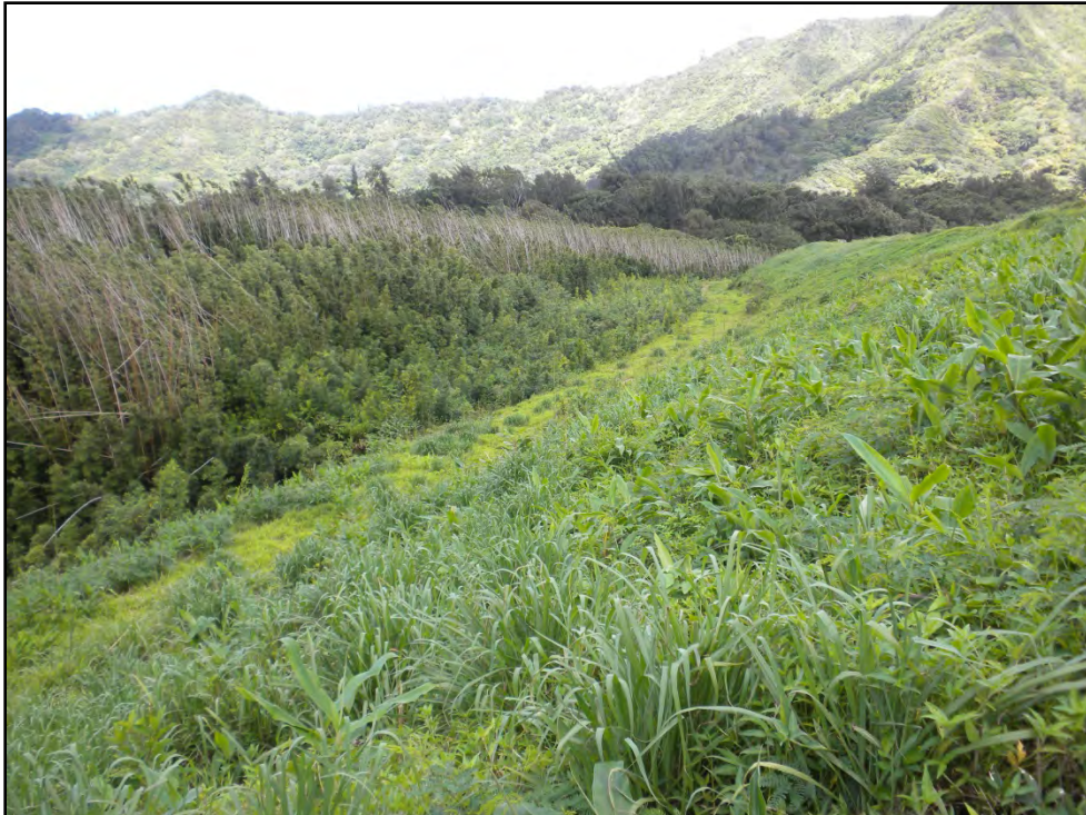
Figure 51. Old access road on downstream side of embankment dam
