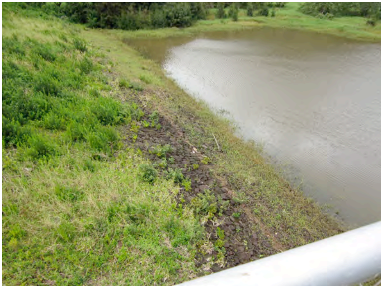
Photo 7: face of dam as seen from bridge to outlet works tower.
