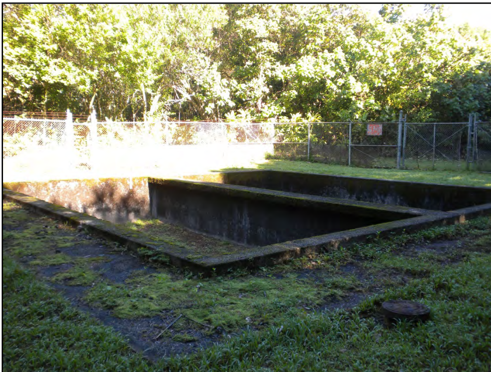
Figure 54. Large vats used for water filtering
