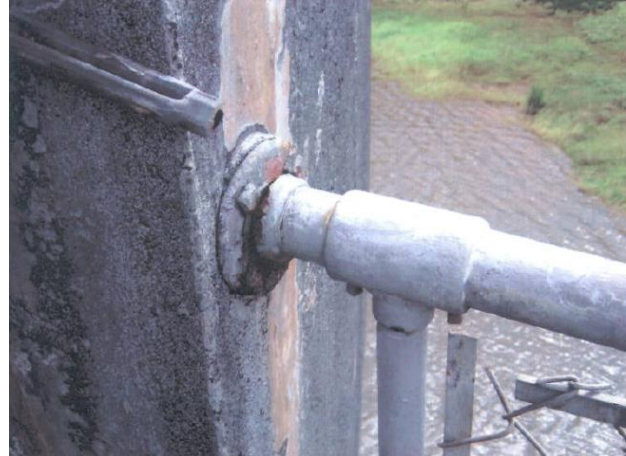
Figure 2-12: Handrail at Intake Tower
