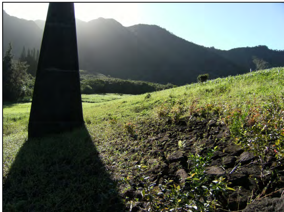
Figure 42. Partial rip-rap surface on the side of the embankment dam
