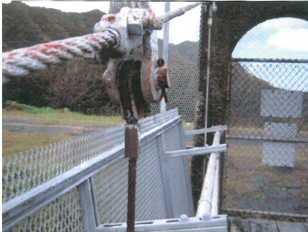
Figure 2-11: Gangway Bolt and Cable.
