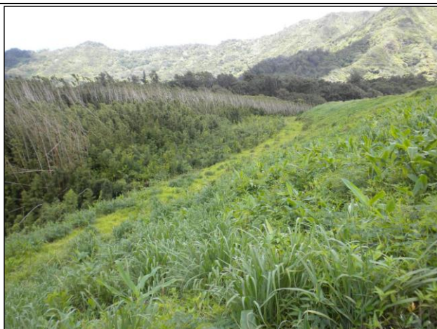
Figure 2-6: Downstream Embankment Face.
