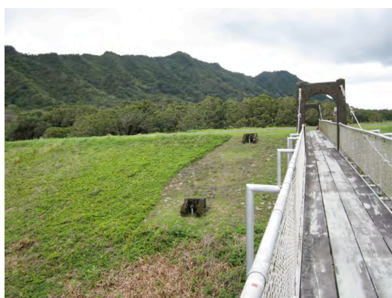
Photo 4: View of dam from intake tower at Nuuanu Reservoir #4. Two monitoring wells on dam are visible.
