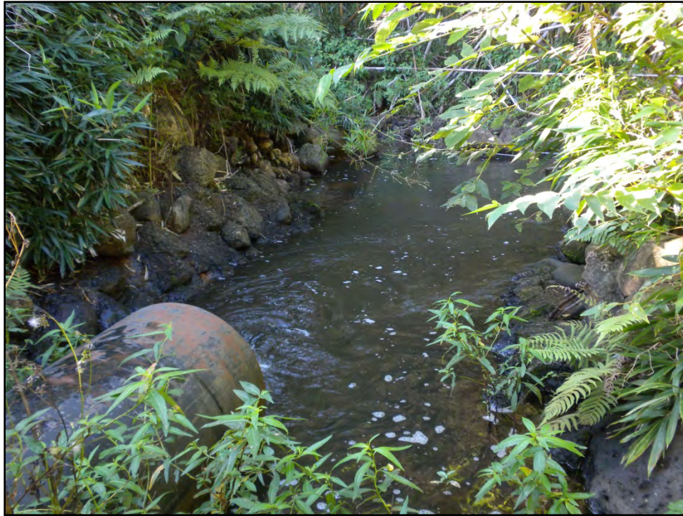
Figure 47. End of 24-inch outlet pipe draining into a shallow stream
