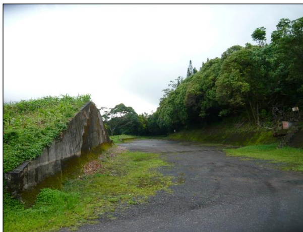
Figure 2-8: Spillway at Dam Crest.
