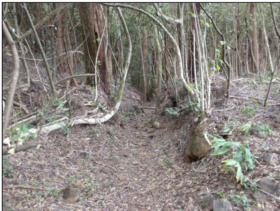
Figure 37. Ditch cut into the natural ground surface
