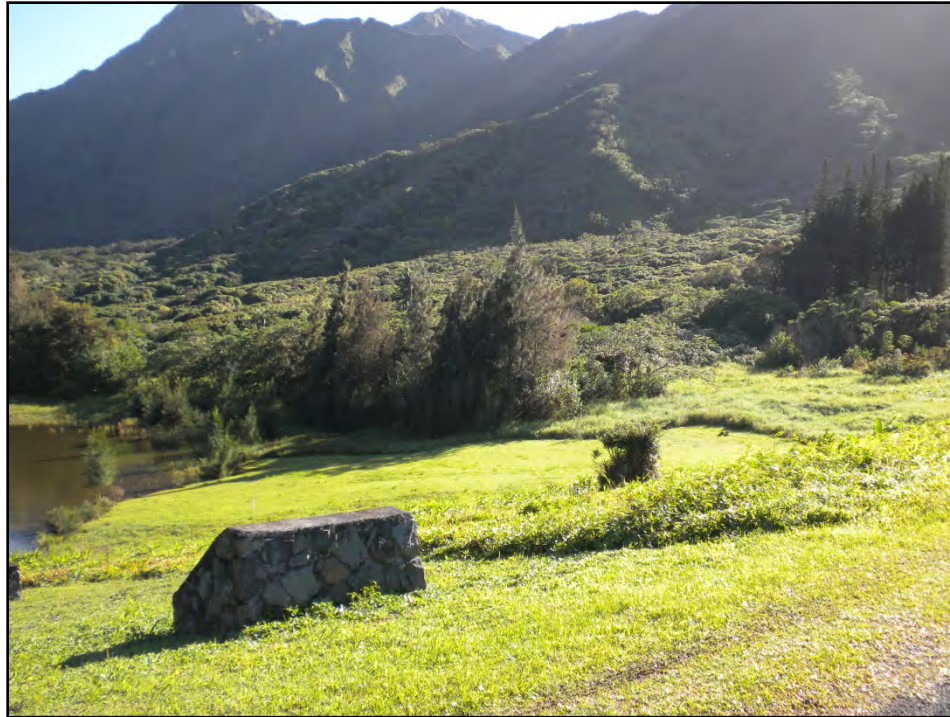
Figure 43. Beginning of spillway to the southeast of the reservoir
