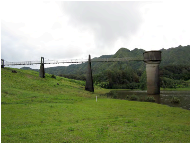
Photo 3: Side view of suspended bridge and outlet works tower.
