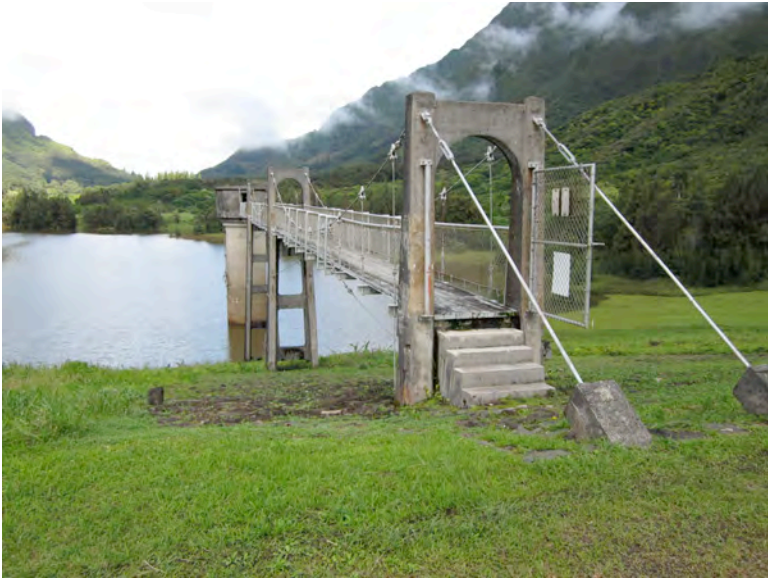
Photo 1: Intake tower at Nuuanu Reservoir #4.
