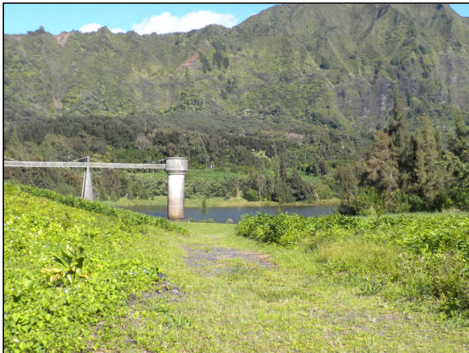
Figure 44. Continuation of spillway to the east of the reservoir
