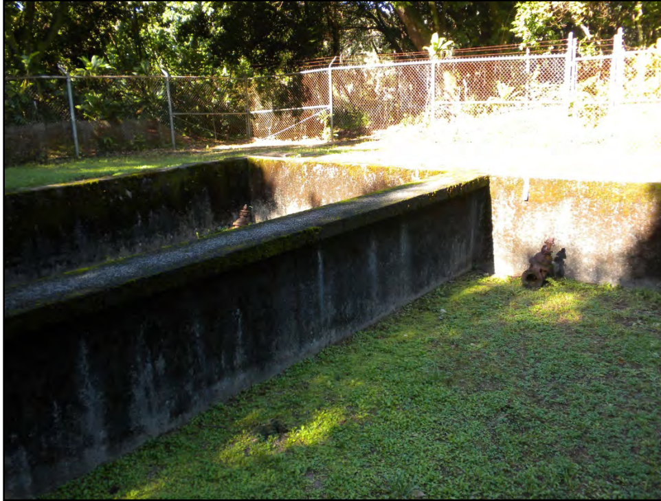
Figure 55. Close-up of water filtering vats, showing valves in the side walls of each vat
