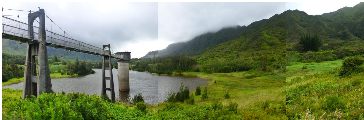
Figure 2-4: Intake Tower and Reservoir Basin Looking Towards the Pali (east).
