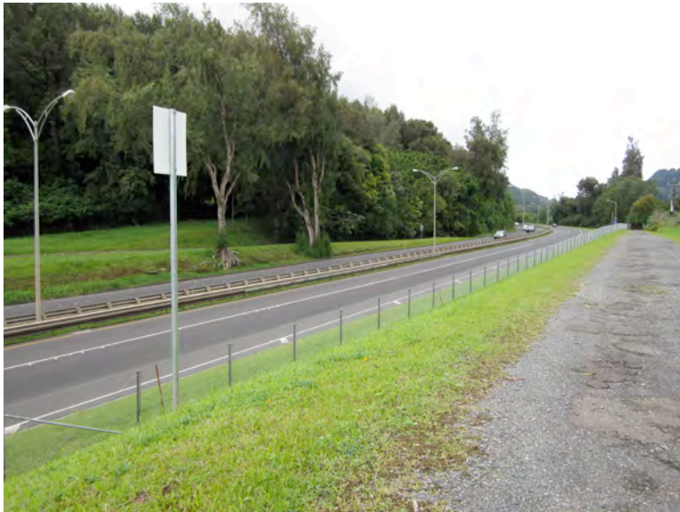
Photo 1: Access road from Pali Highway leading to Nuuanu Reservoir #4.
