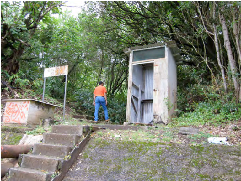
Photo 9: Stairway leading from paved spillway toward sand filter area at Nuuanu Reservoir #4.
