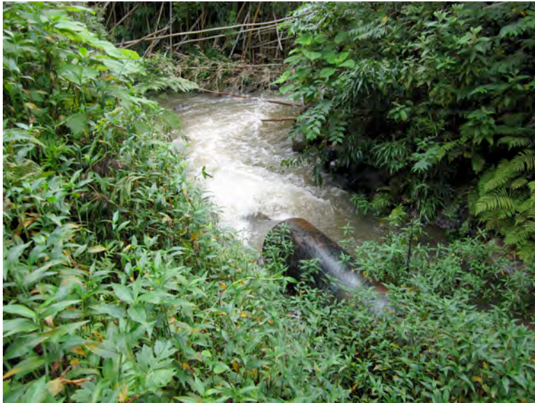
Photo 5: Outflow from outlet pipe at toe of Nuuanu Reservoir #4 dam.
