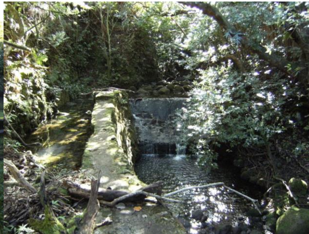
Figure 3-14: Concrete Wall at Lulumahu Stream
