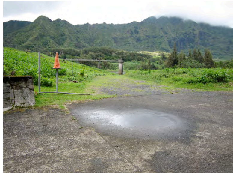
Photo 8: View from dam spillway looking toward reservoir at Nuuanu Reservoir #4.
