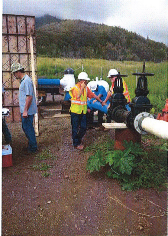
Figure 2: Pictures showing the sound-proofing baffle around diesel engine, piping, and right-angle drive with water level sounder and measuring tube.
