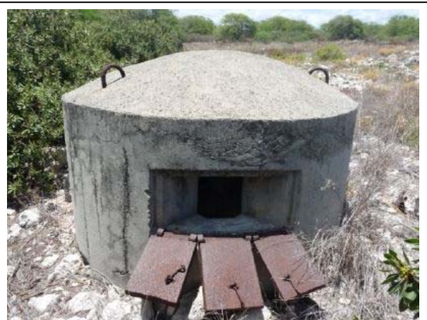
Concrete World War II structures, including pillboxes (above), were discovered within the Kalaeloa Unit during restoration activities. The USFWS continues to conduct activities, plans, and programs aimed at preserving and enhancing these resources as well as all historic and cultural properties. Photograph courtesy of the USFWS.
