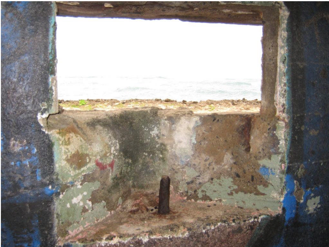
Figure 14. Site 7261 gun mount, view to north
