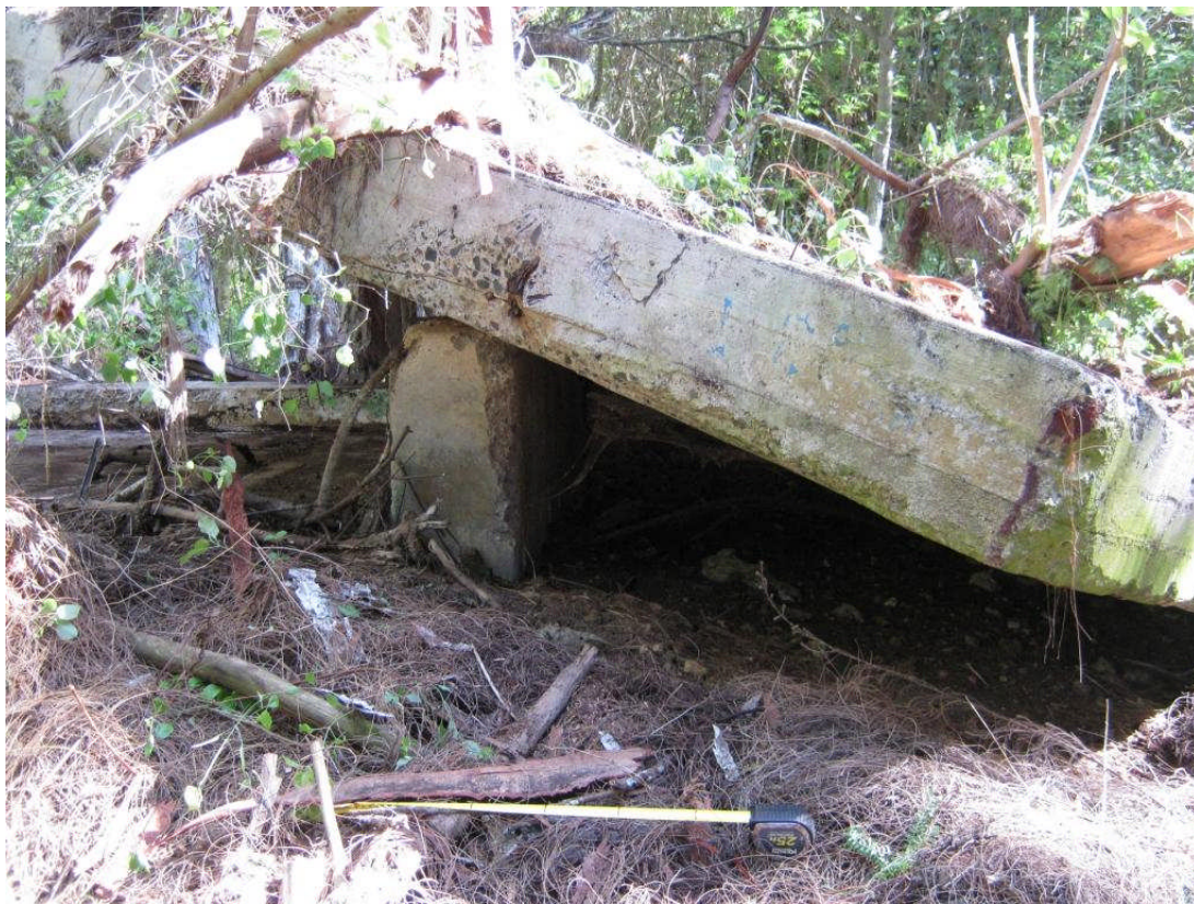
Figure 61. Site 7281 concrete structural remnant, view to south
