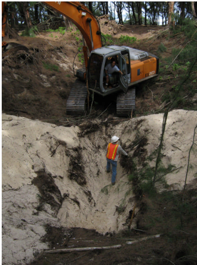
Figure 39. Area C, Sand Pit 1 showing mechanical excavation, view to south
