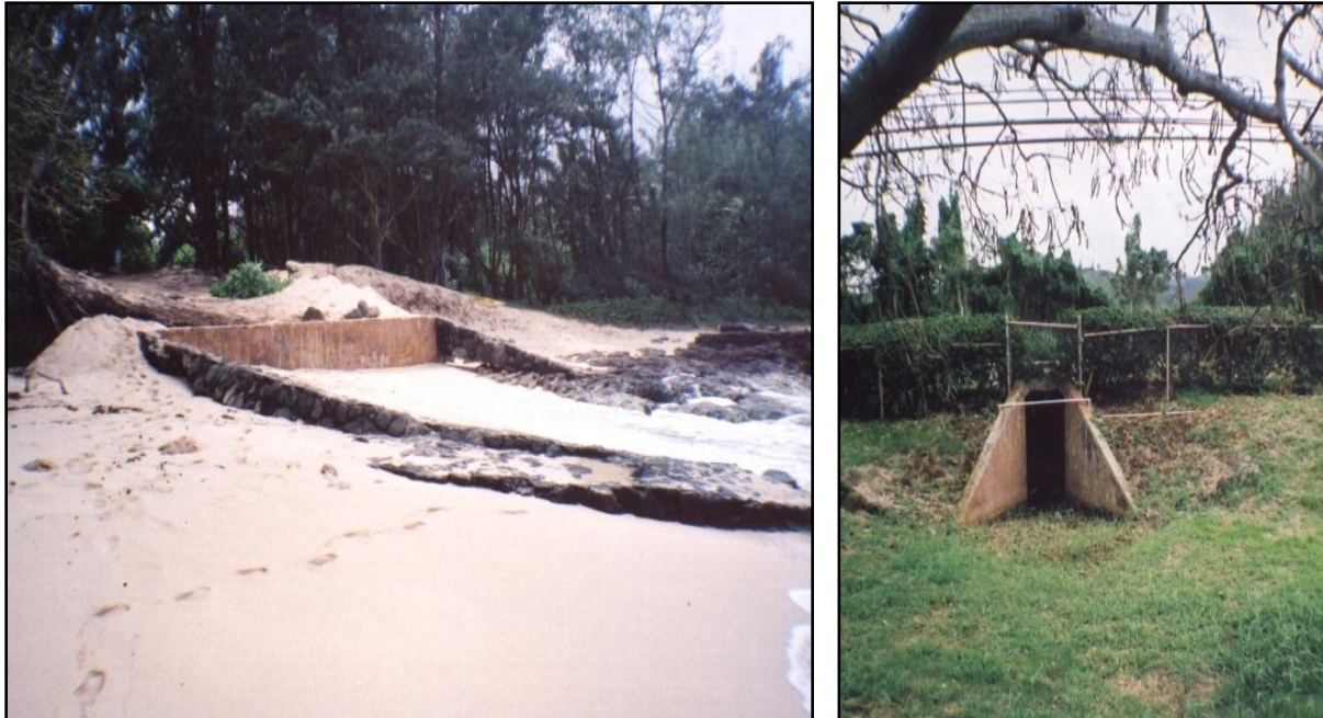
Figure 4-2. West Main Drain Outlet (above) to Turtle Bay is typically buried in sand when not actively flowing. The small channel under Kamehameha Highway (right) limits flow to the West Main Drain from mauka of the highway.
