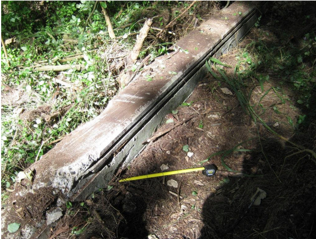
Figure 60. Site 7281 concrete structural remnant, view to northeast
