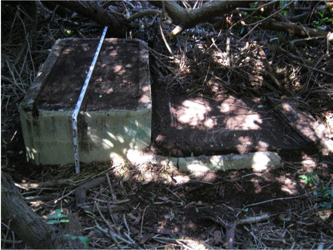
Figure 79. Concrete platform at Site 7284, Feature D, view to west
