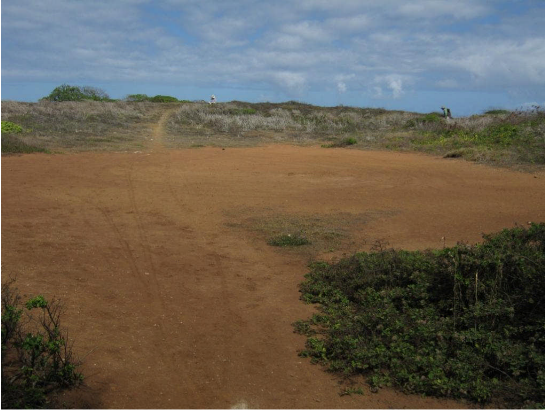
Figure 18. Site 7264 revetment, view to north
