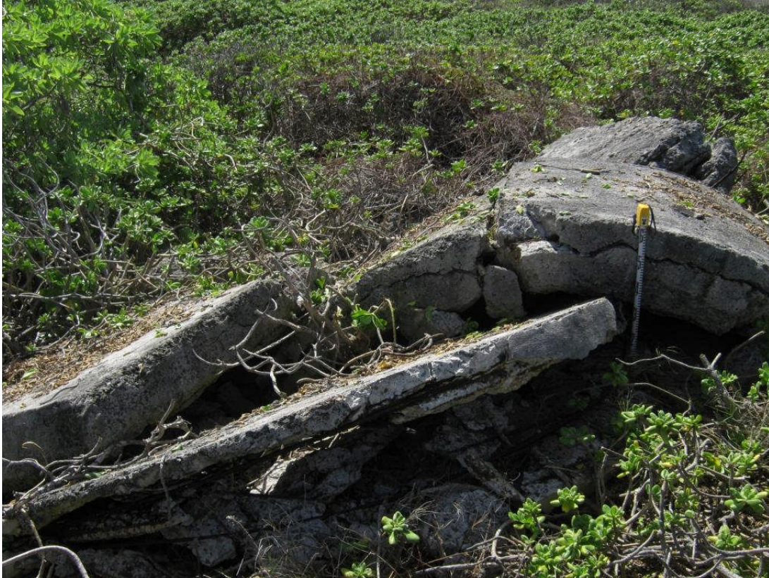
Figure 21. Site 7268 concrete structural remnant, view to south
