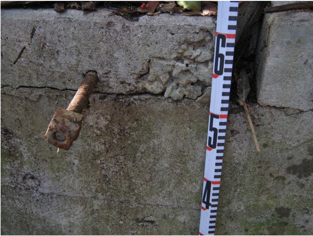
Figure 75. Bolts on side of Site 7284, Feature C, view to southwest
