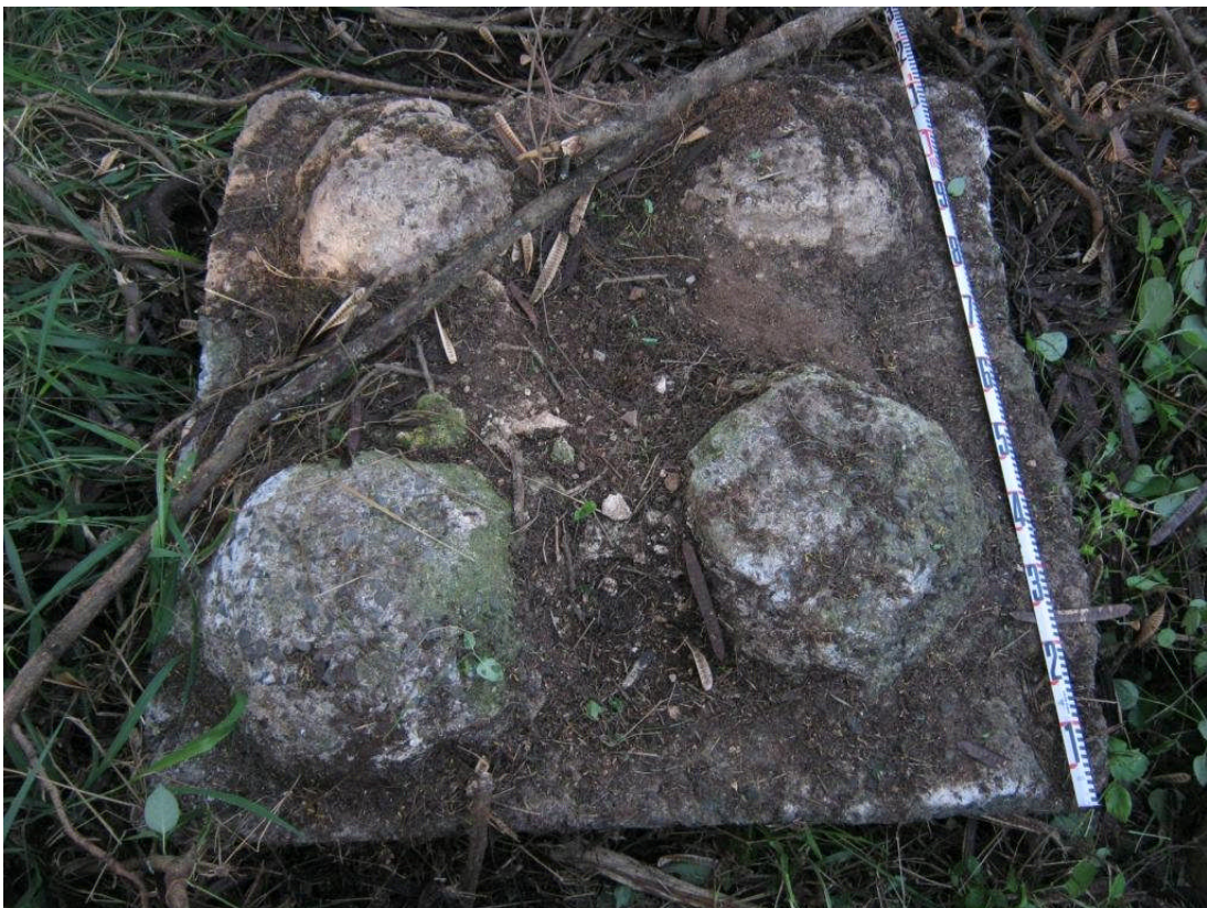
Figure 72. Site 7284, Feature B concrete pad with projections, view to northwest
