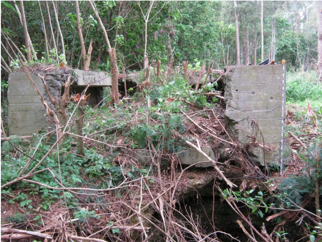
Figure 49. Site 7278 concrete structure, view to northwest
