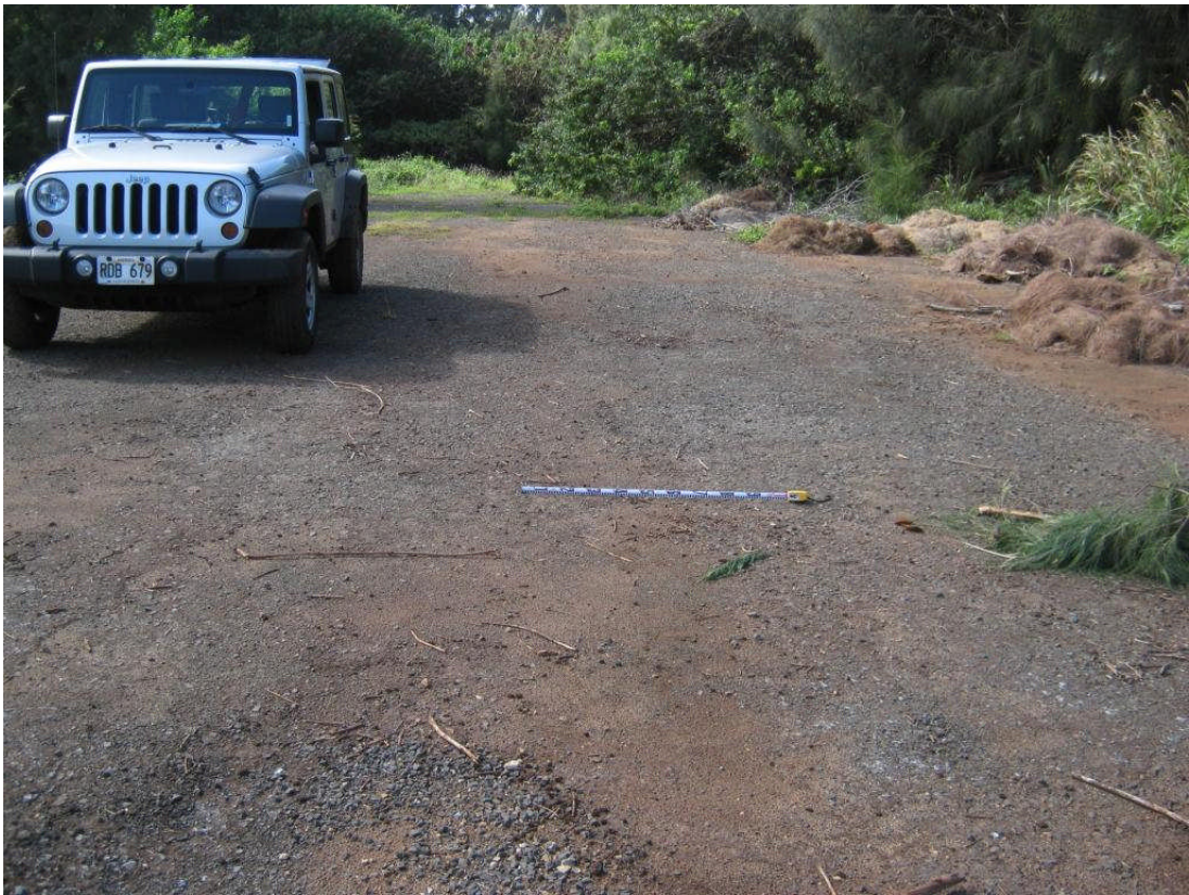
Figure 82. Site 7286 asphalt pavement, view to west
