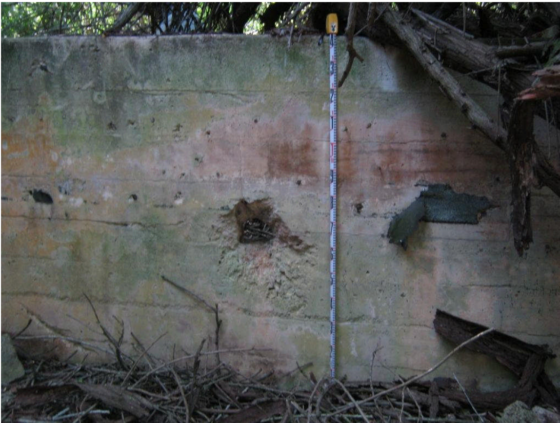
Figure 78. Site 7284, Feature D wall, view to northeast
