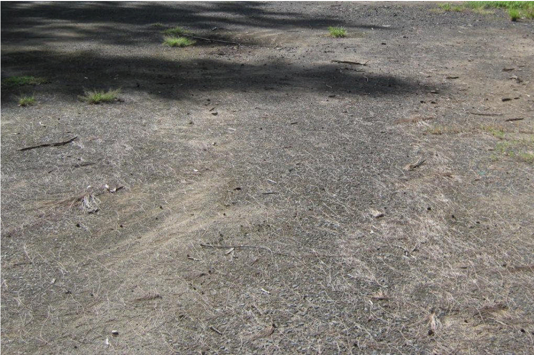
Figure 26. Site 7271 asphalt area, view to east
