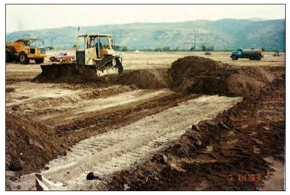
Photo 9.24, 07/14/93 Removal of pockets of organic material from the landfill subgrade.
