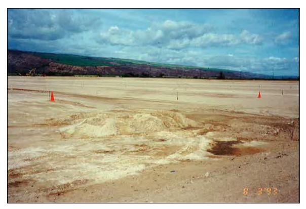
Photo 13.01, 08/03/93 Looking southwest across fine graded portion of the landfill subgrade.
