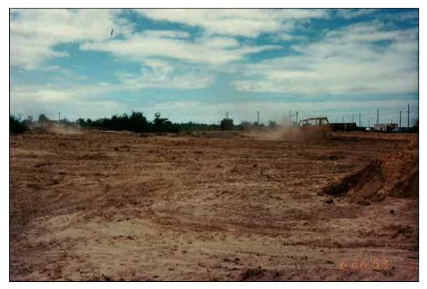
Photo 1.18, 06/26/93 Dozers clearing, grubbing and stripping at the north end of the site.
