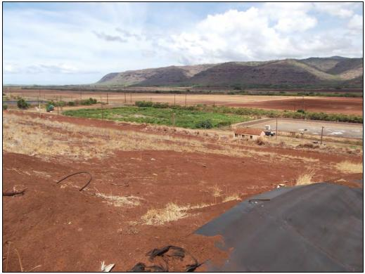
Looking mauka from the crest of the current landfill. Leachate pond visible on right; stormwater infiltration basin (heavily vegetated) visible on left. Former "linear mound" ran between the two and under the leachate pond location, and is no longer present.
