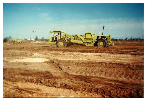
Photo 7.20, 07/10/93 Scrapers loading silty material containing wood debris and hauling it to waste area.
