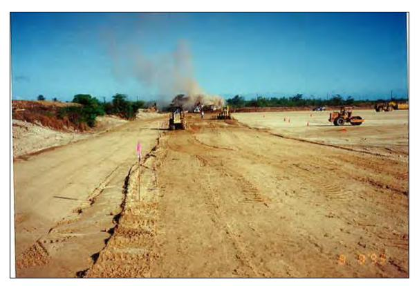
Photo 14.04, 08/09/93 Placement of roadway embankment near station 36+00.
