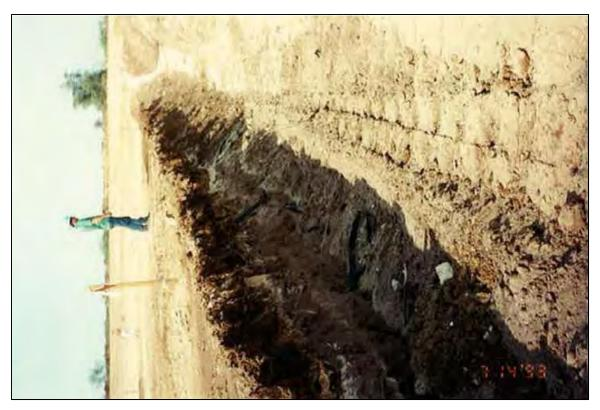
Photo 9.21, 07/14/93 Cut section of area where organic pocket was removed.
