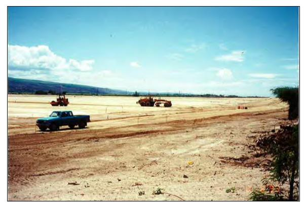
Photo 13.21, 08/06/93 Looking south at fine grading of the landfill subgrade.
