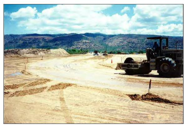
Photo 13.19, 08/06/93 Looking east at the placement of roadway embankment station 42+00 to 51+00.
