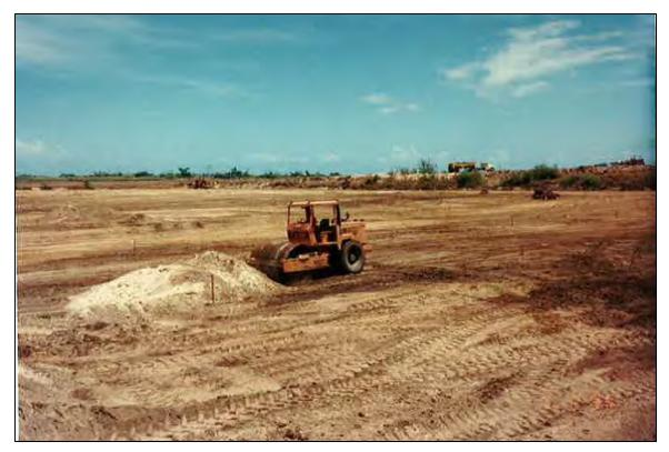
Photo 4.18, 07/02/93 Roller compacting subgrade prior to placement of landfill embankment.
