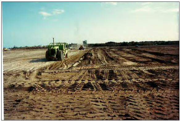
Photo 3.24 06/30/93 Excavation of the landfill to subgrade.
