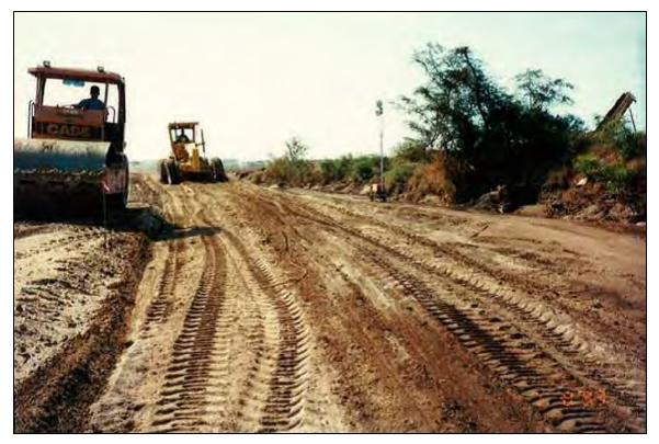
Photo 6.09, 07/08/93 Grader removing unsuitable material from roadway.
