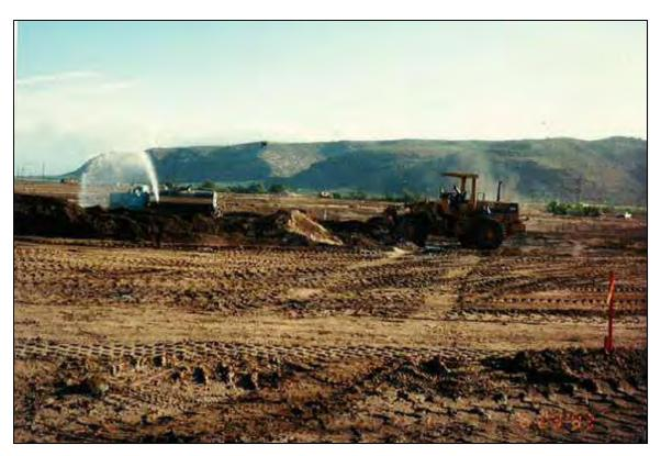
Photo 3.02 6/29/93 Stockpiling of organic material removed from landfill subgrade.
