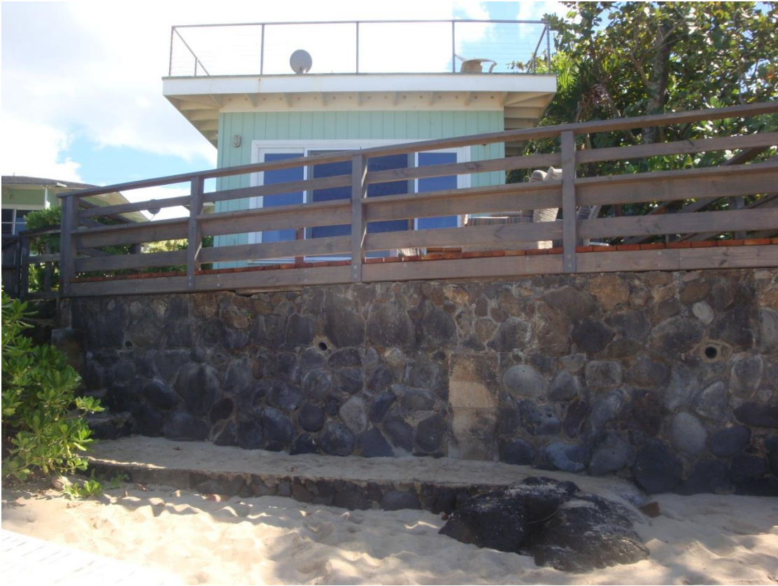
Figure 7: Close up of Moss Rock Retaining Wall
