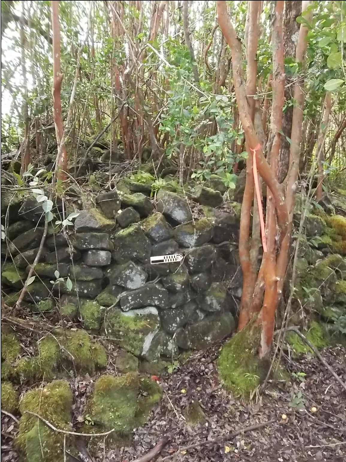
Figure 28: Photograph of Site 29905 Looking West.
