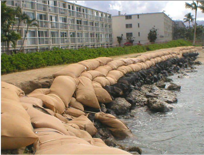
Figure 3-10i. Beach Erosion & Sandbag Revetment at North End in November 2005 (Courtesy of Jeanne Marx)
