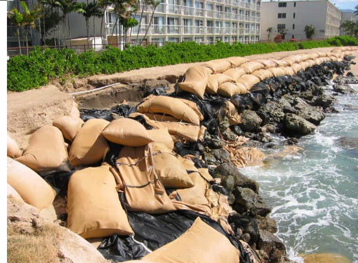
Figure 3-10j. Beach Erosion & Sandbag Revetment at North End in January 2006
