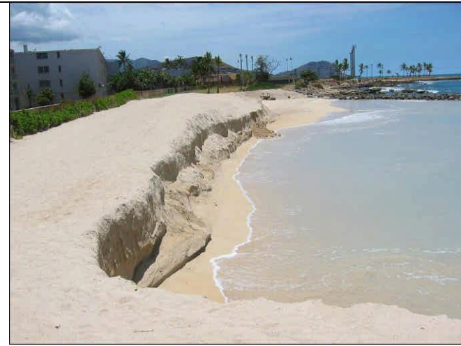
Figure 3-10h. Beach Nourishment Shortly after Placement
