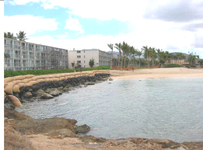
Figure 3-10b. View from North End in 2006; Sandbag Revetment
