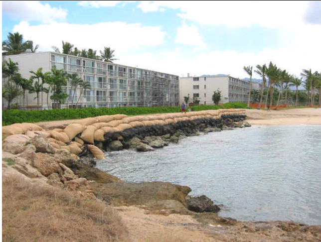
Figure 3-10a. View from North End in 2006; Sandbag Revetment
