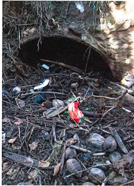
Figure 4. Culvert under a footpath over Kailua Stream appears to hold water on a regular basis (November 2013).
