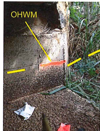
Flag Culvert Right
