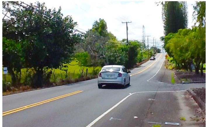
5 Haihai Street (westbound) near Hilo Municipal Golf Course Parking Entry Showing the Adequate Sight Distance
