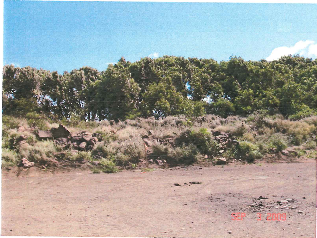
Photograph No. 7 At the Waiale Road and East Waiko Road Intersection Looking South Towards Waikapu Stream
