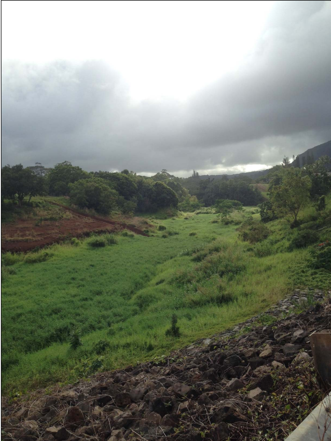
Photo 3-4: View from Kainahola Road looking upstream. Photo taken from near the reservoir outlet. Note rip rap in foreground. This rock was placed during the dam repair project. Road cut on the left mid-field of the photo is the approximate location of the south embankment of the replacement dam.
