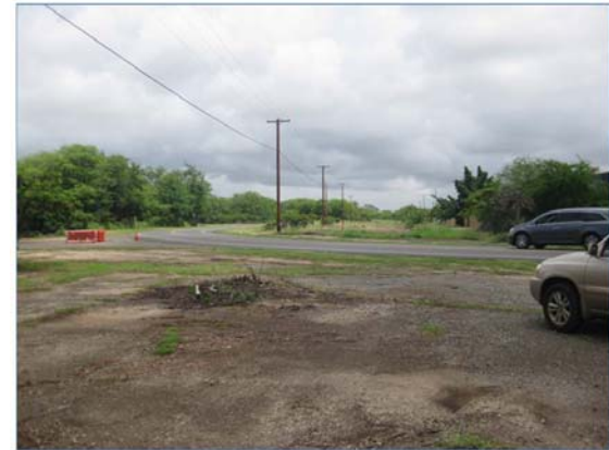
Fig. 9. Above Geiger Road, the vegetation of the Corridor is dominated by bare ground and weedy grasses.
