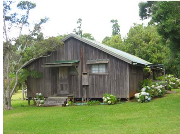
Photo 4-3 “Kōkeʻe Rustic” Board and Batten Architecture Rice Flat, (TMK: 1-4-04: 19)
