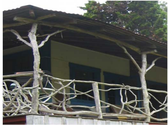
Photo 7-3 ‘Ōhi‘a Wood Railing Detail TMK: 1-4-02: 10
