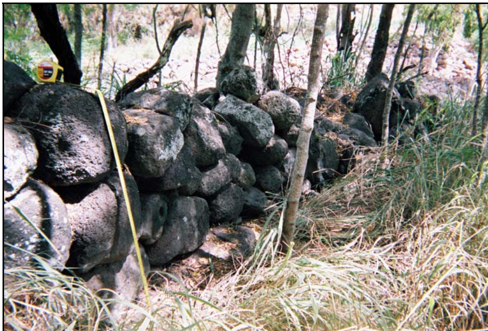
Figure 24. Photographs of portions of the SIHP # 50-80-07-6896 stone wall (above, view to west) (below, view to southwest)
