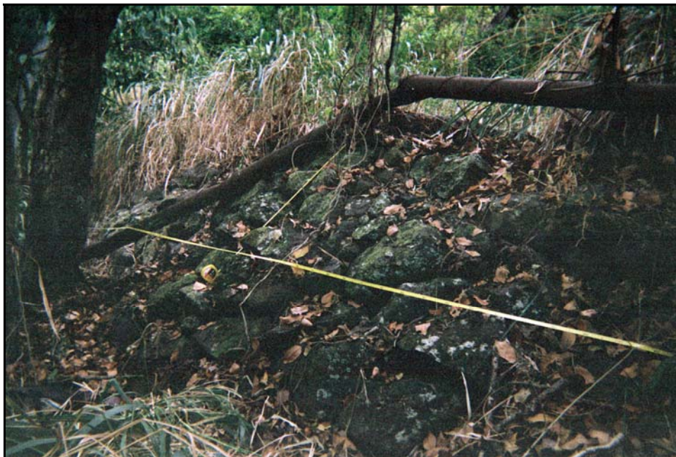
Figure 21. Photograph of SIHP # 50-80-07-6895 Feature G retaining wall, view to southeast
