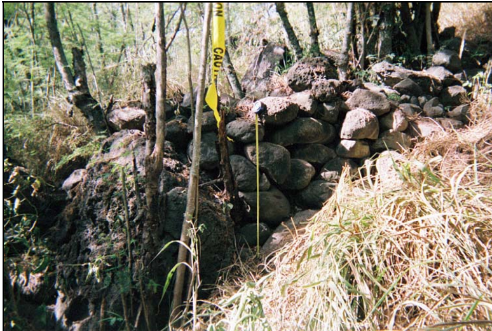
Figure 20. Photograph of SIHP # 50-80-07-6895 Feature F terrace, view to north
