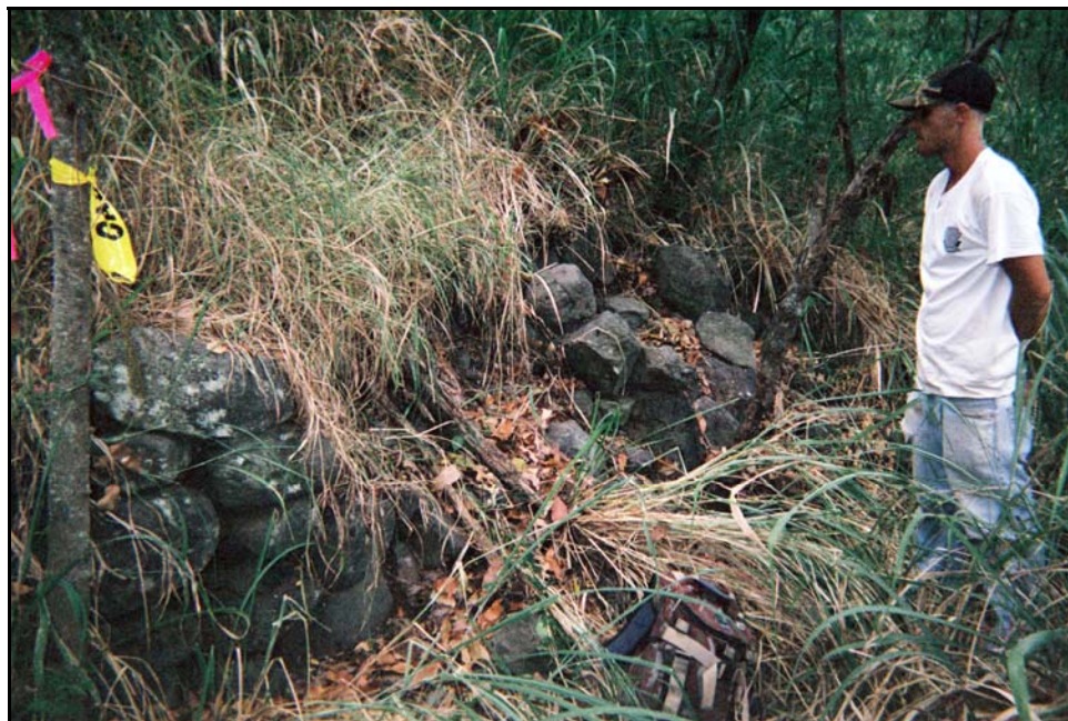
Figure 16. Photograph of SIHP # 50-80-07-6895 Feature C retaining wall, view to southeast
