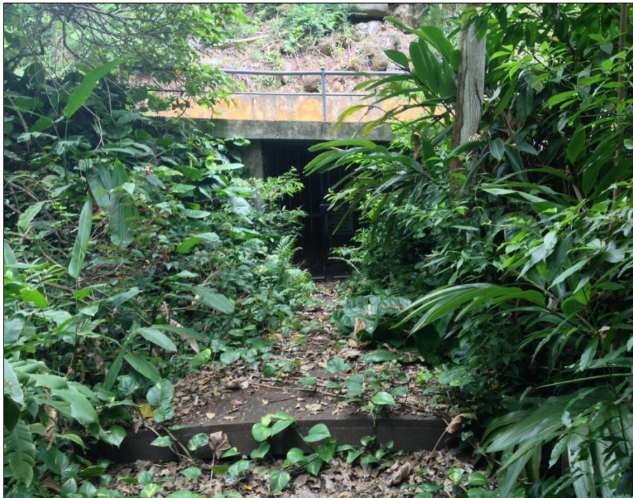
Figure 16. Glover Tunnel Portal
