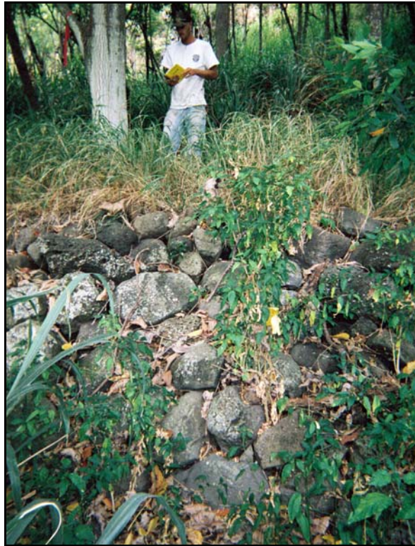
Figure 15. Photograph of SIHP # 50-80-07-6895 Feature B retaining wall, view to southeast
