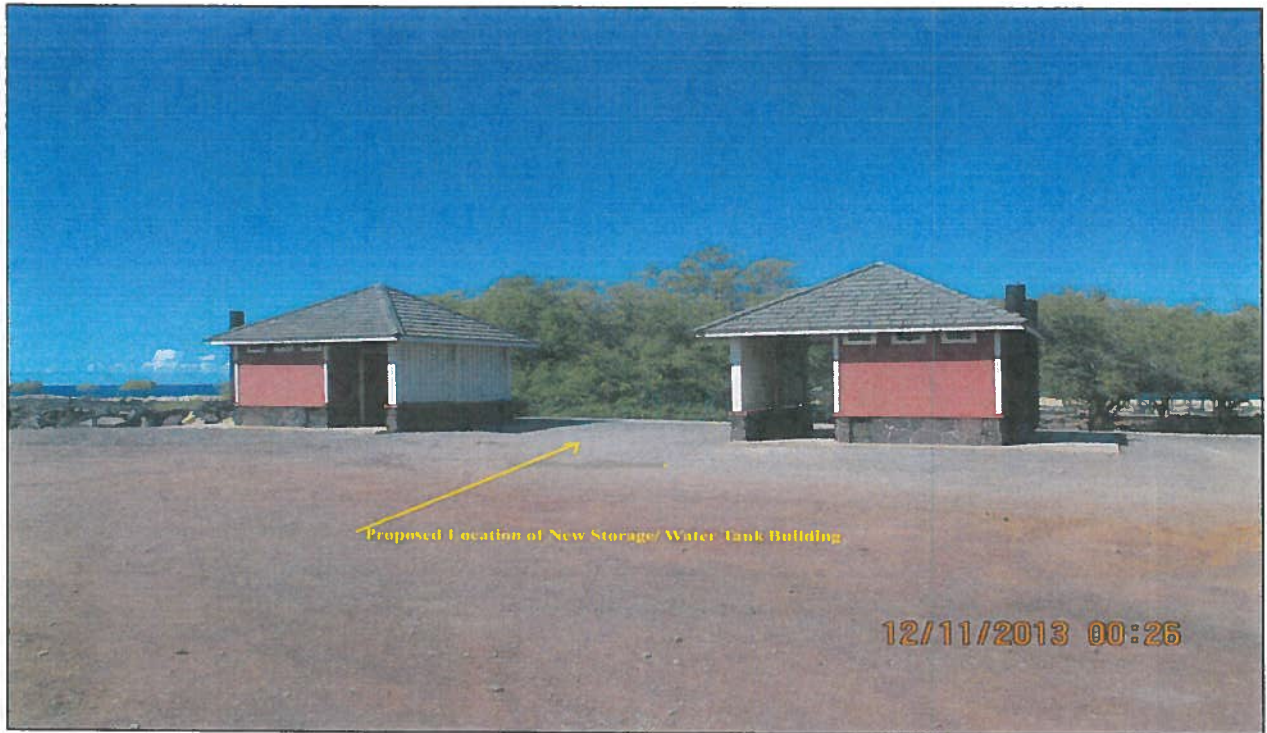
PHOTO 1. Proposed location of new storage/water tank building to be built between the existing comfort station buildings as shown. View is to the west ( makai ).
