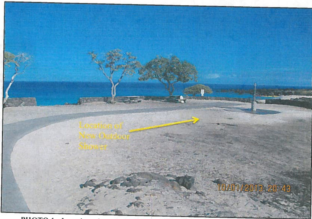
PHOTO 1: Location of the new outdoor shower on the mauka side of the existing walkway, view to the NW.
