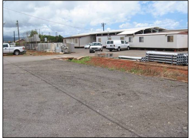
Photo 10: View of DFM/Department of Transportation Services (DTS) Portable Buildings.
