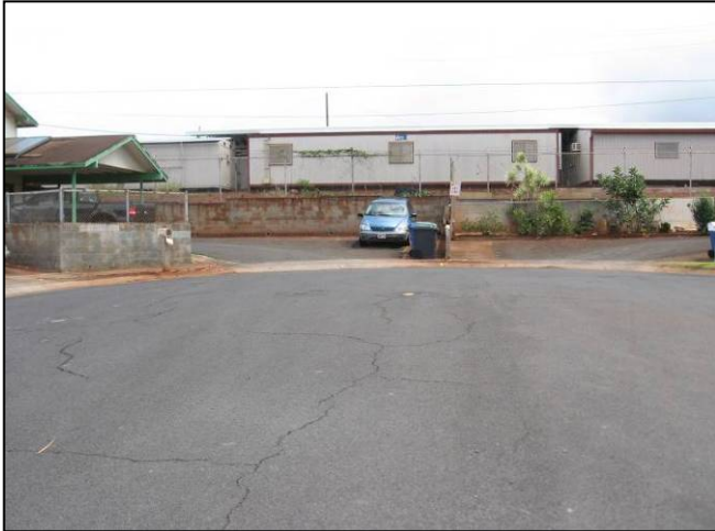
Photo 11: View of DFM/DTS Portable Buildings From Adjacent Residential Subdivision (Kanaeha Place).
