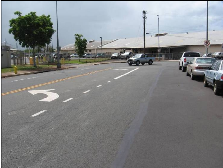
Photo 1: View of Department of Parks and Recreation (DPR) Warehouse from Makolu Street.
