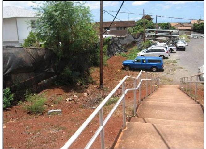
Photo 12: Stairway Connecting Upper to Lower Area. Residential Area to Left.
