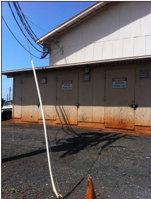
Photo 7: Outside of DPR Chemical Section.
