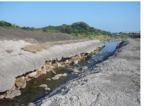
Eroded bank toe at river station 54+00.
