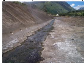
**Low-flow stream channel** (picture taken prior to flow restoration).
