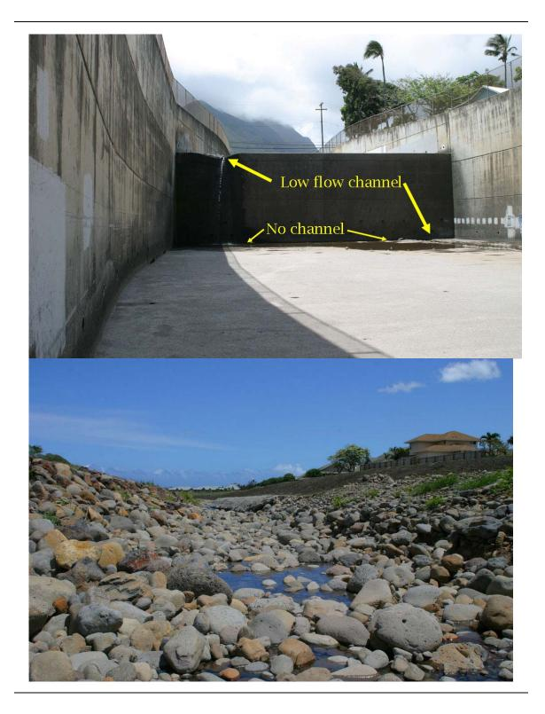
Figure 4a (top). In places, the low-flow channel is not continuous. Figure 4b (bottom). An unlined stream section in the Project area.
