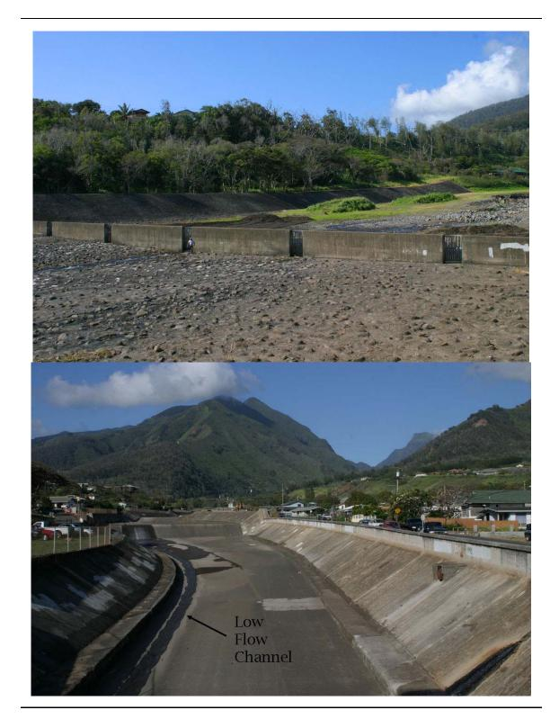
Figure 2a (top). Debris basin (note biologist in white shirt for scale). Figure 2b (bottom). Concrete channel of 'Īao Stream showing low flow channel.
