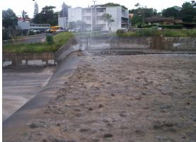
Drop structure and diversion feature (picture taken prior to flow restoration).
