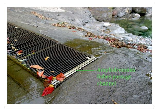
Figure 3. Fish passage structure at 'Īao Tunnel intake on 'Īao Stream.
