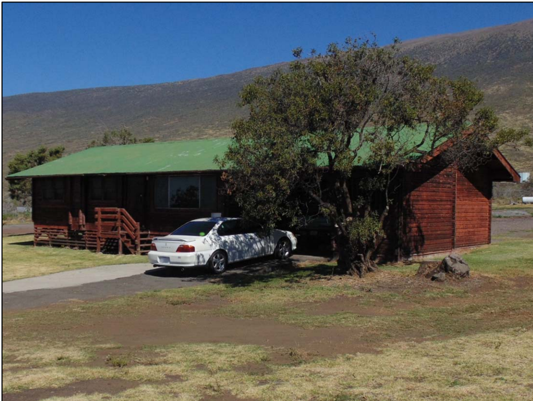
Figure 23. Caretaker's cabin built with prefabricated Pan-Abode logs, view to northwest.
