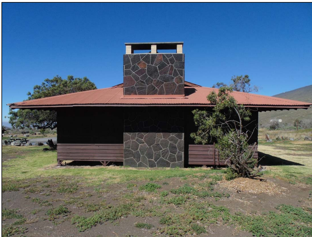
Figure 21. Lava veneer chimney and Douglas fir siding on the Dining/Recreation Hall, view to the west.
