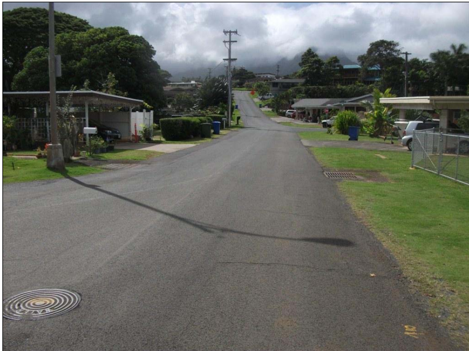
Figure 26. Kahanahou Circle (front section) and Lilipuna Road (back section), view southwest toward junction with Lilipuna Place; note manhole in center of roadway (CSH photograph)
