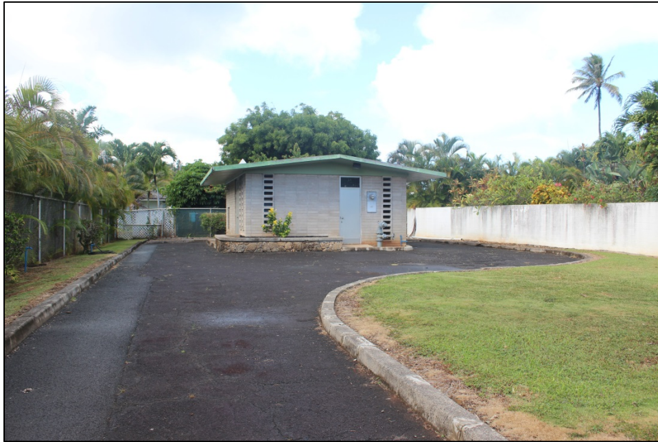
Kahanahou Wastewater Pump Station as seen from Ka Hanahou Place.
