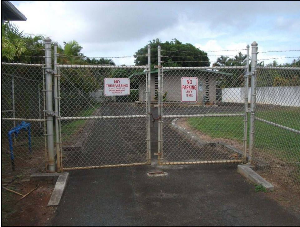
Figure 21. Kahanahou Wastewater Pump Station, eastern end of project area, view to northwest (CSH photograph)
