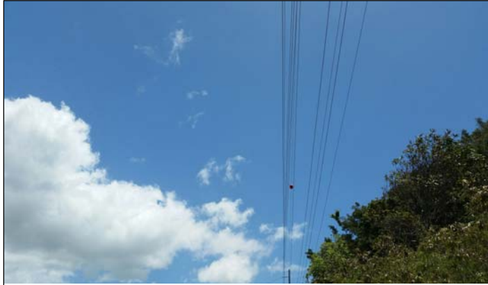
View of KIUC power lines bisecting the project site.
