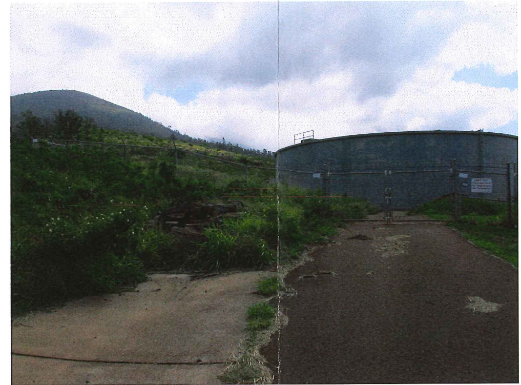
East View of 1 mg water tank
