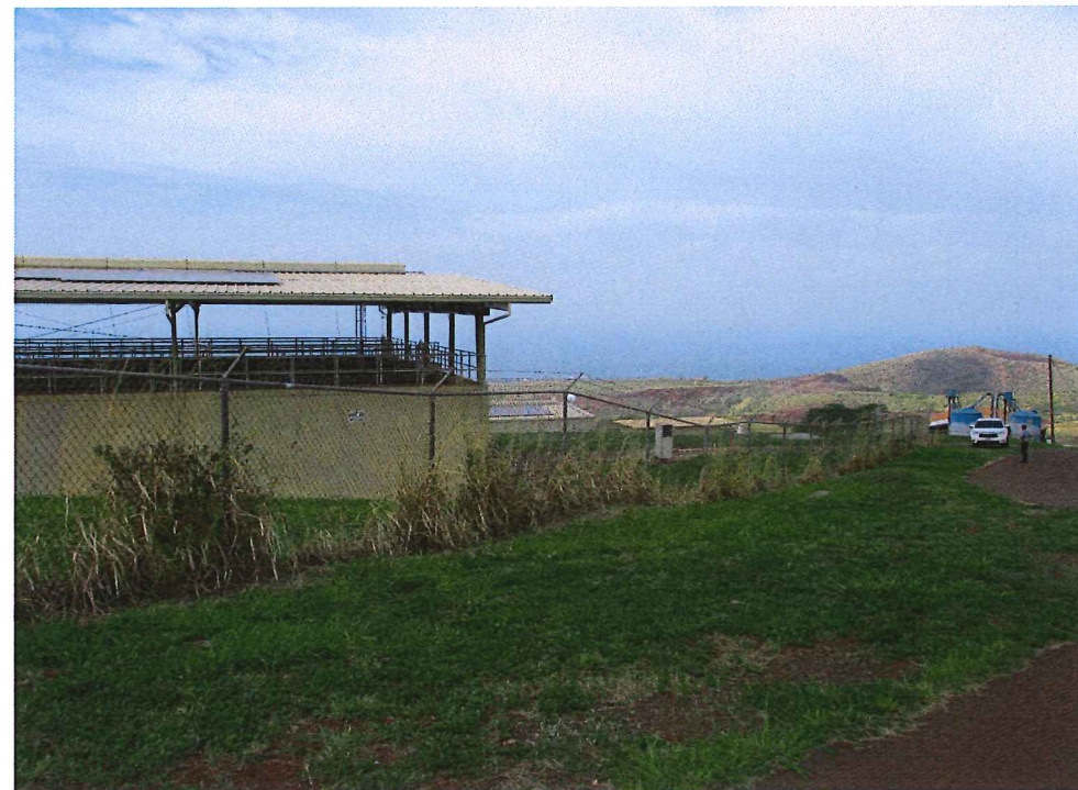
West view of sedimentation basin
