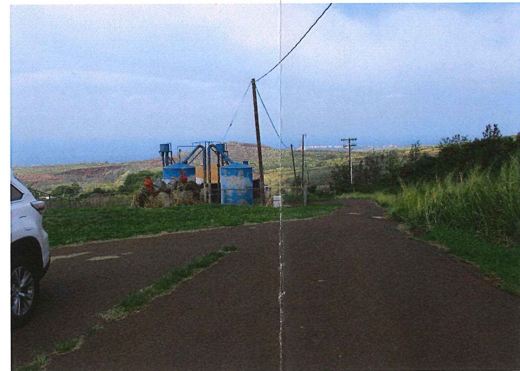
Northwest view of utility poles along DWS access road
