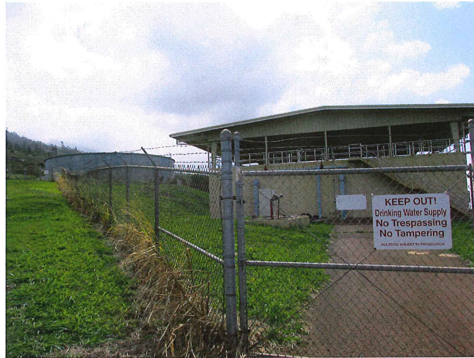
Southeast view of 1 mg water tank and sedimentation basin
