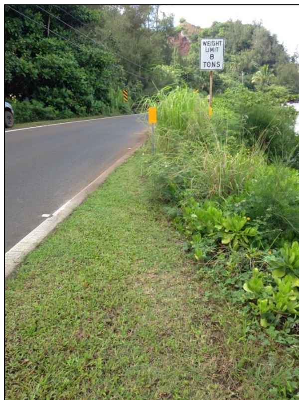
Figure 4. Waikoko Bridge survey area ornamental landscaping and ruderal vegetation.
