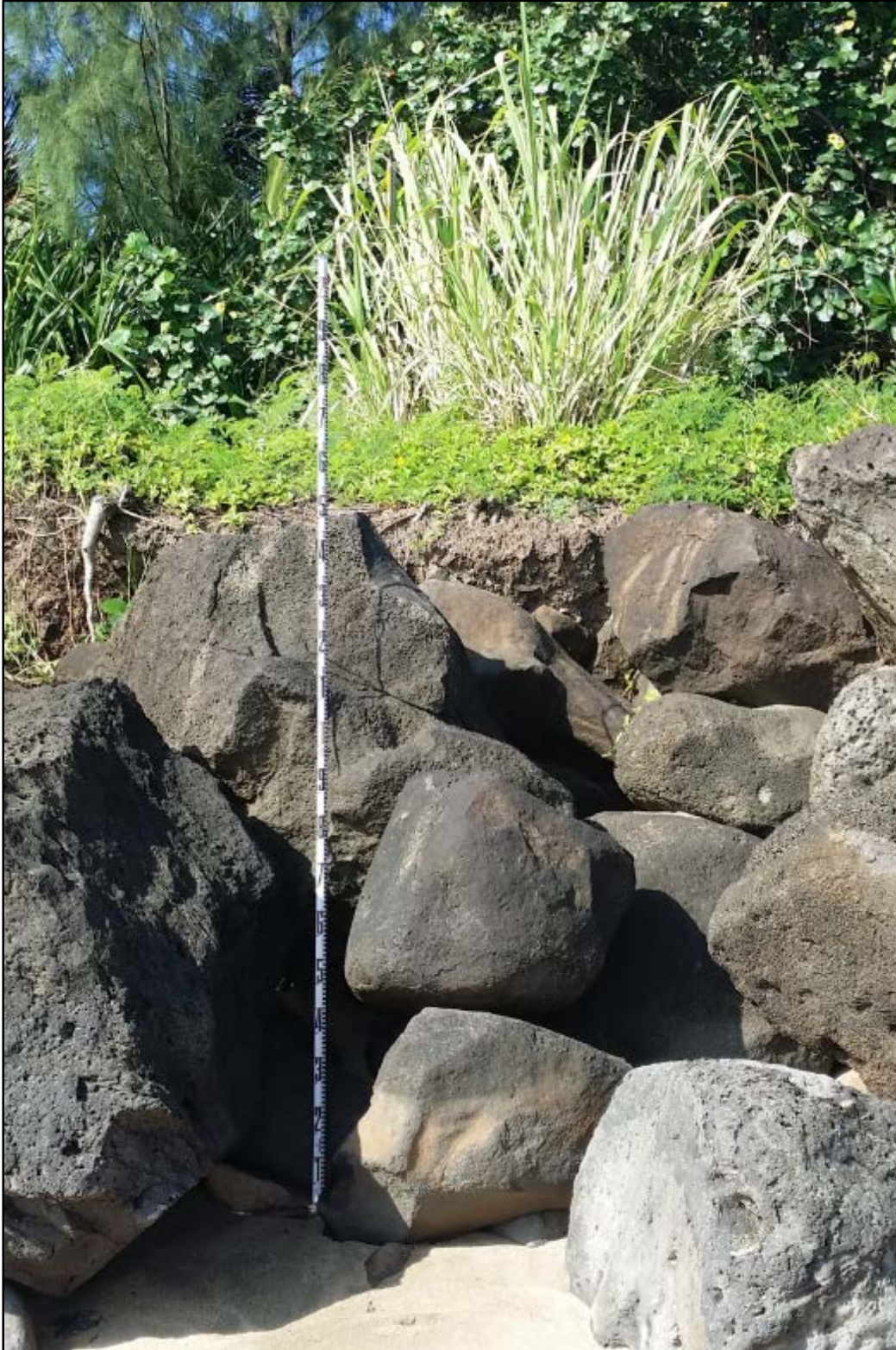
Figure 67. Southern portion of SIHP # 50-30-03-2298, basalt boulder base course of the Waikoko Stream Bridge, view to north
