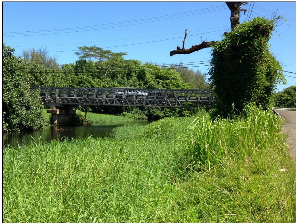
Figure C6. Wainiha Bridge 3 taken from the mauka east bank.
