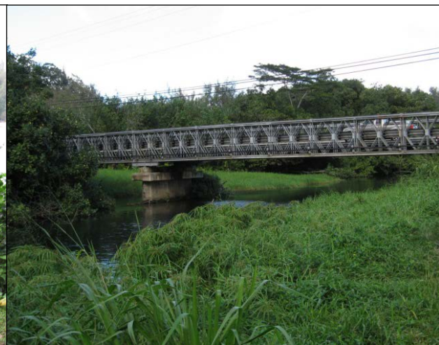
Existing ACROW Bridge 3
