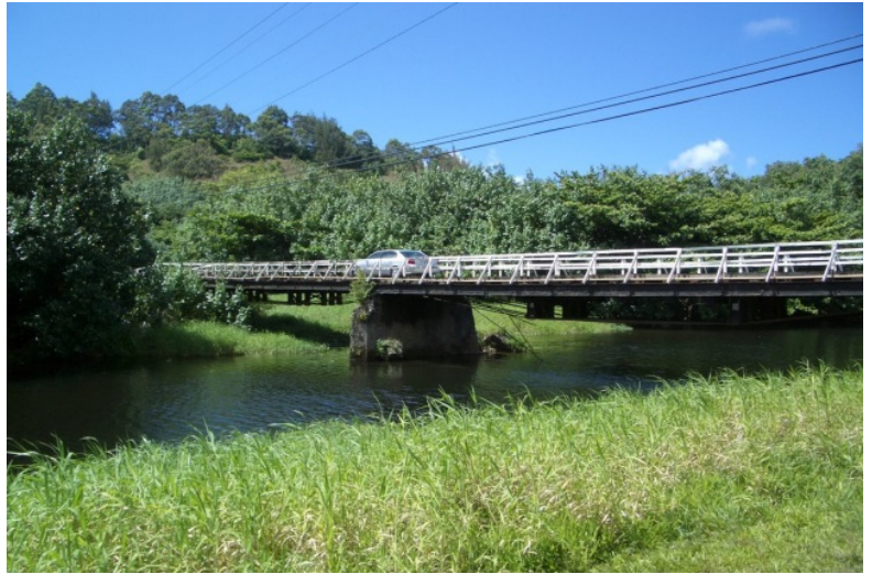
Historic pre-ACROW Bridge 3
