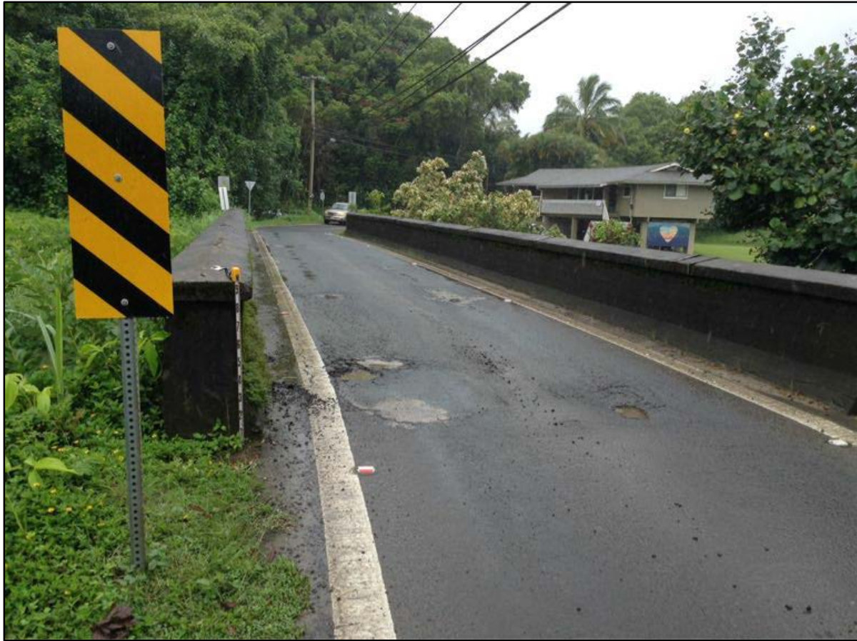
Figure 46. SIHP # 50-30-03-2296, Wai'ole Stream Bridge, profile view to north
