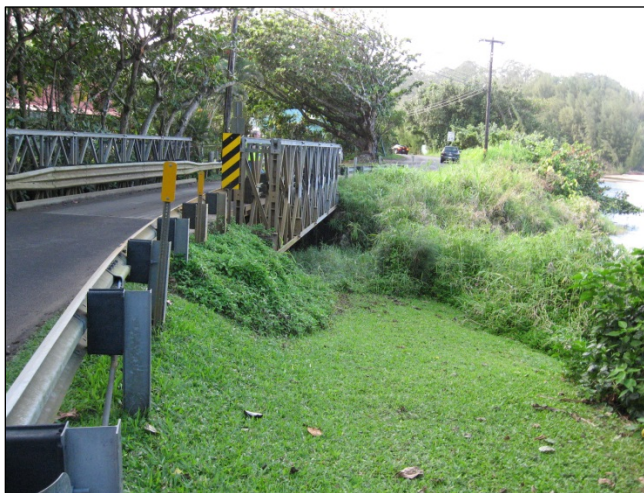
Existing ACROW Bridge 1
