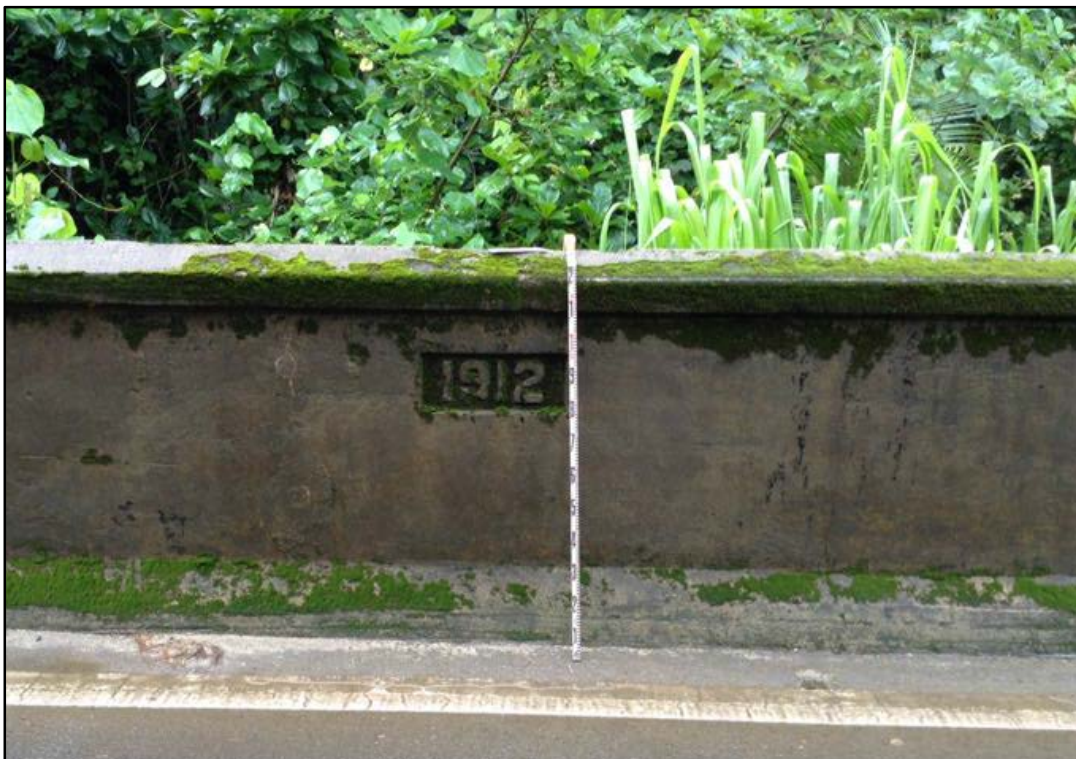
Figure 56. SIHP # 50-30-03-2297, the Waipā Stream Bridge, showing concrete stamped “1912,” view to west
