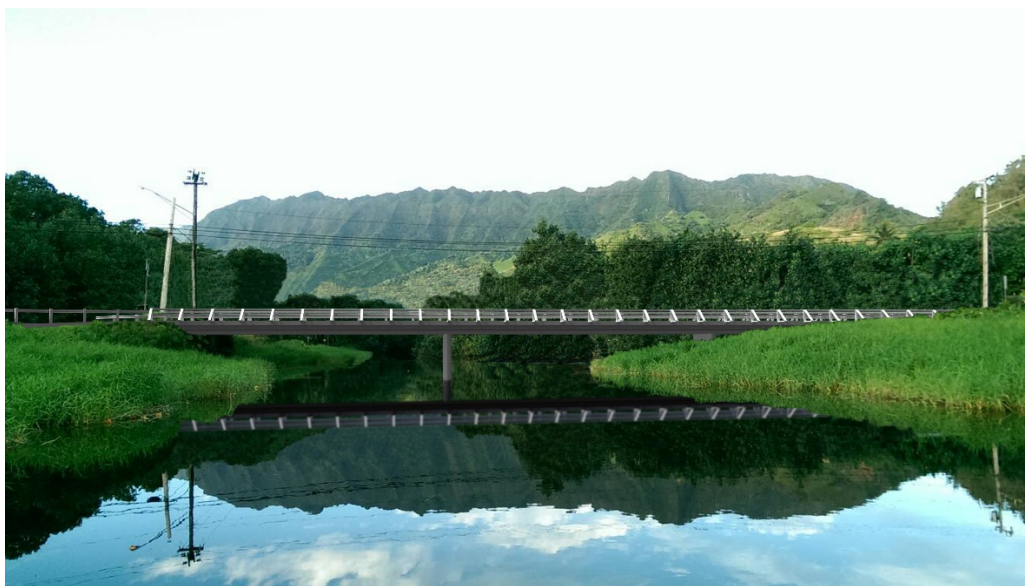
Simulation 2: Simulation of proposed Wainiha Bridge 3 from Wainiha River looking southwest (upstream)
