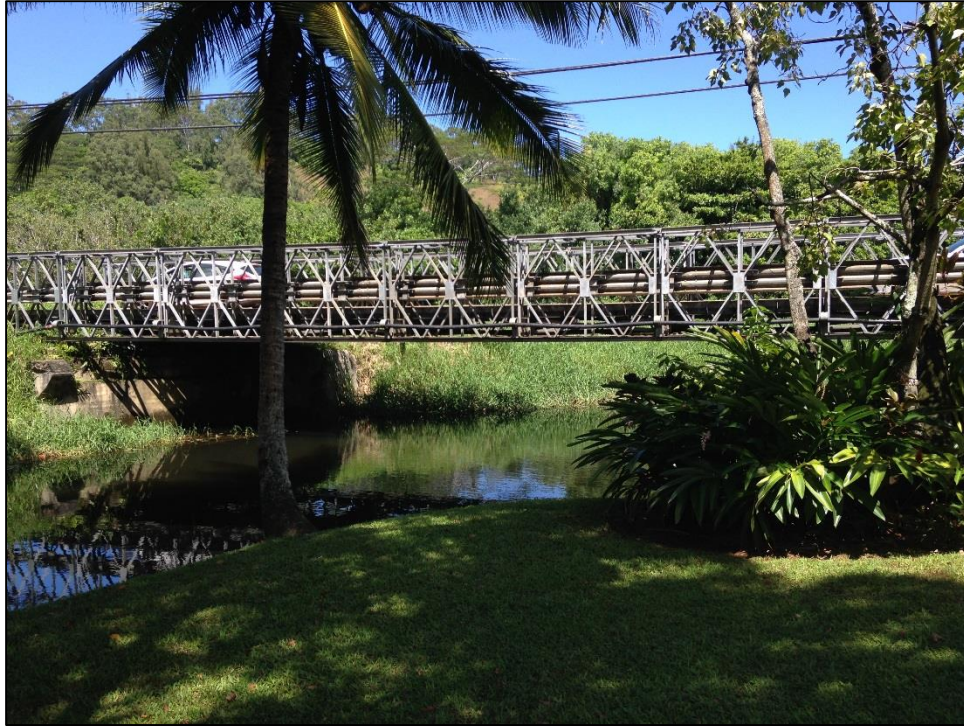
Figure C5. Wainiha Bridge 2 taken from the mauka east bank.
