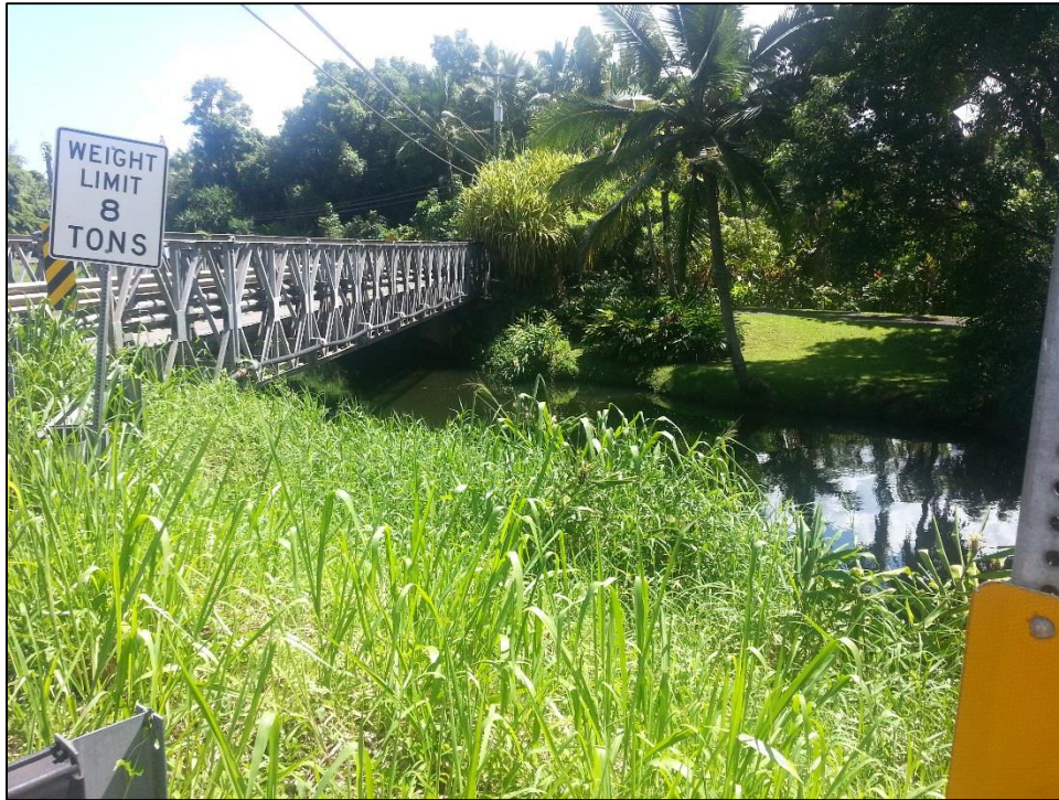
Figure 7. Wainiha Bridges 2 & 3 survey area (mauka/upstream side).
