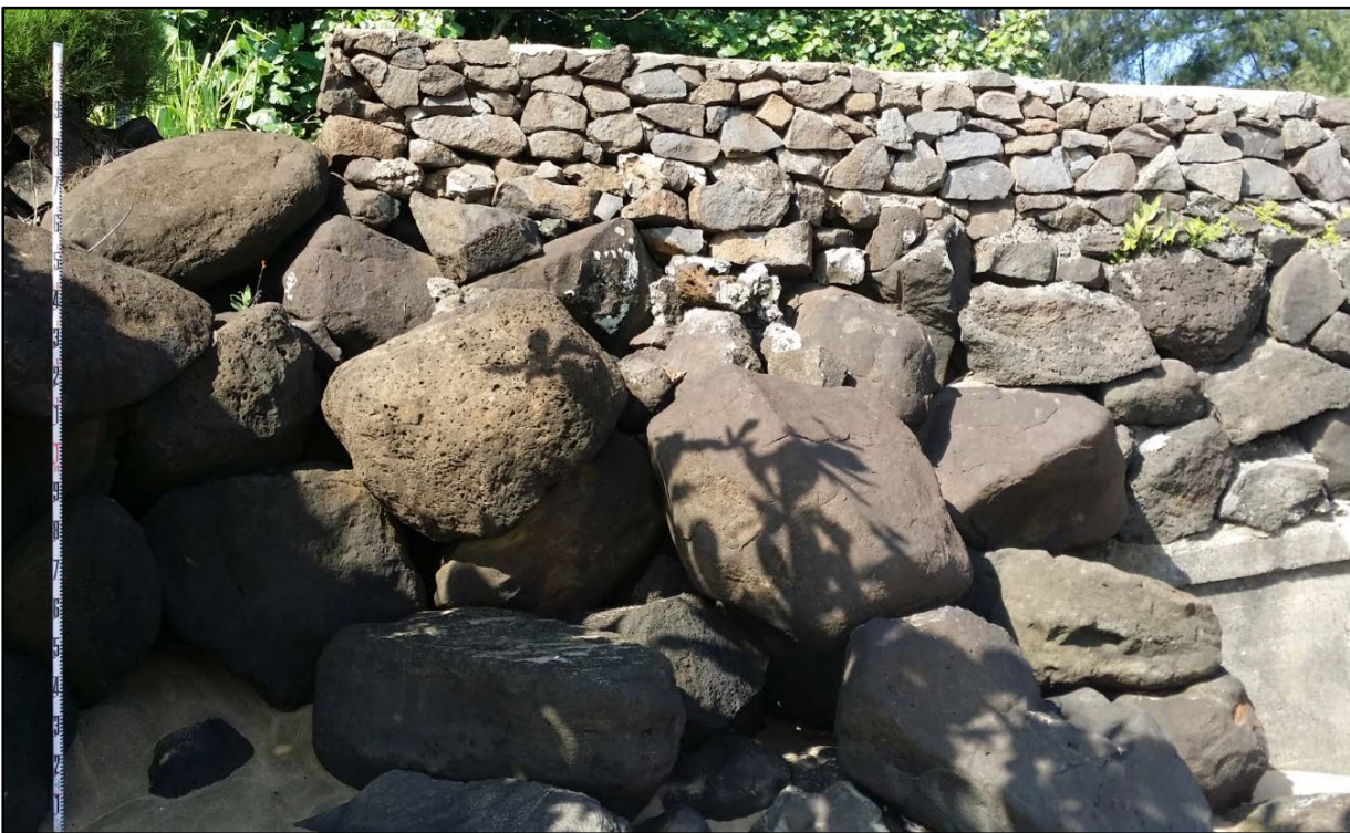
Figure 61. SIHP # 50-30-03-2298, the Waikoko Stream Bridge, profile view to west of the southern terminus of the bridge's makai face; note the successive courses of stacked and mortared basalt (one through eight)
