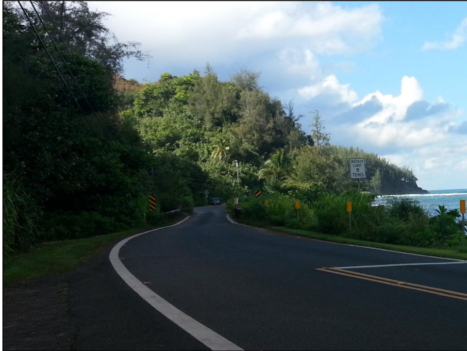
Figure C3. Waikoko Bridge at road, taken from the south.
