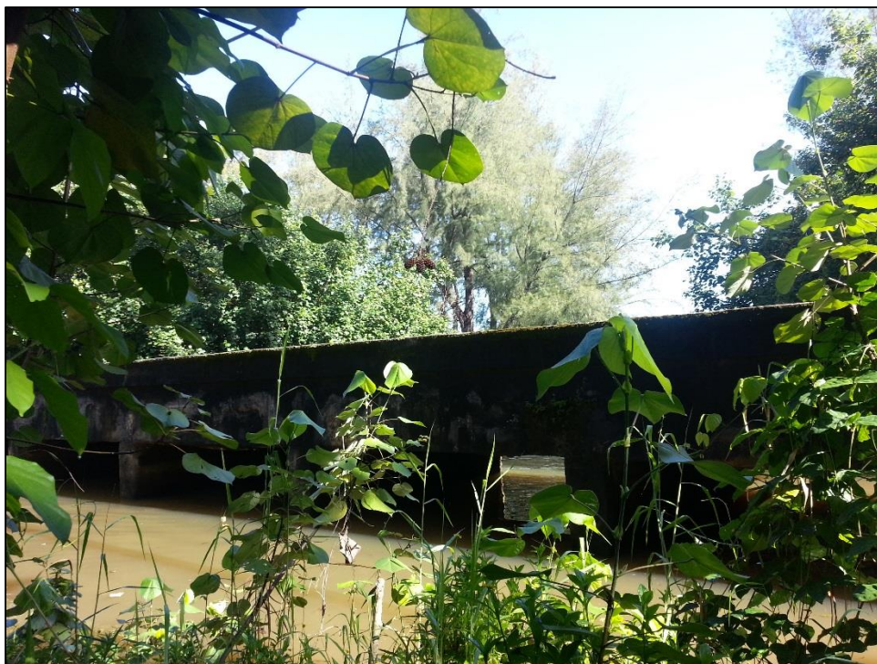
Figure C2. Waipā Bridge taken from the mauka east bank.
