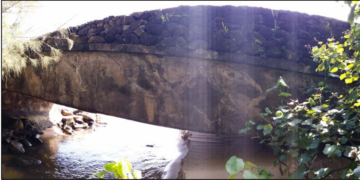
Figure 62. SIHP # 50-30-03-2298, the Waikoko Stream Bridge, general view to northeast of the bridge's mauka face; note approximately five courses of basalt boulders mortared on top of the concrete portion of the bridge damaged in the 1946 tsunami
