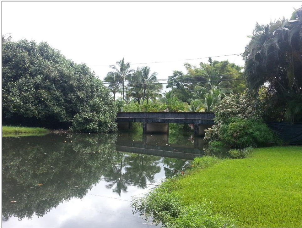
Figure C1. Wai'oli Bridge taken from the makai west bank.
