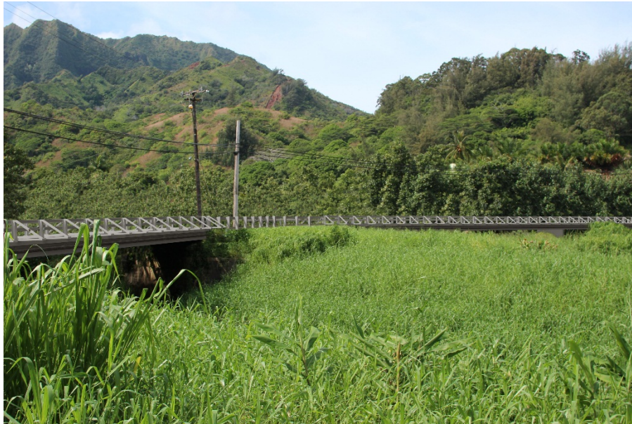
Simulation 1: Simulation of proposed Wainiha Bridge 2 (on the left) and Bridge 3 (on the right) from the highway near the eastern approach to Bridge 2 looking west toward Hā'ena (from Kūhiō Highway)
