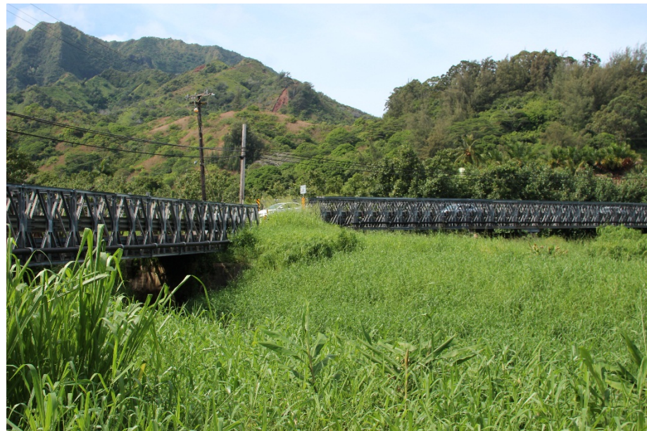
Photo 3: View of existing Wainiha Bridge 2 (on the left) and Bridge 3 (on the right) from the highway near the eastern approach to Bridge 2, makai side, looking west toward Hā'ena (from Kūhiō Highway).
