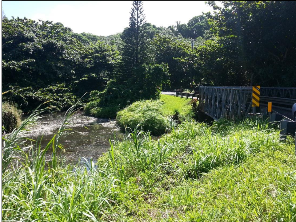
Figure 5. Wainiha Bridge 1 survey area (makai/ downstream side).
