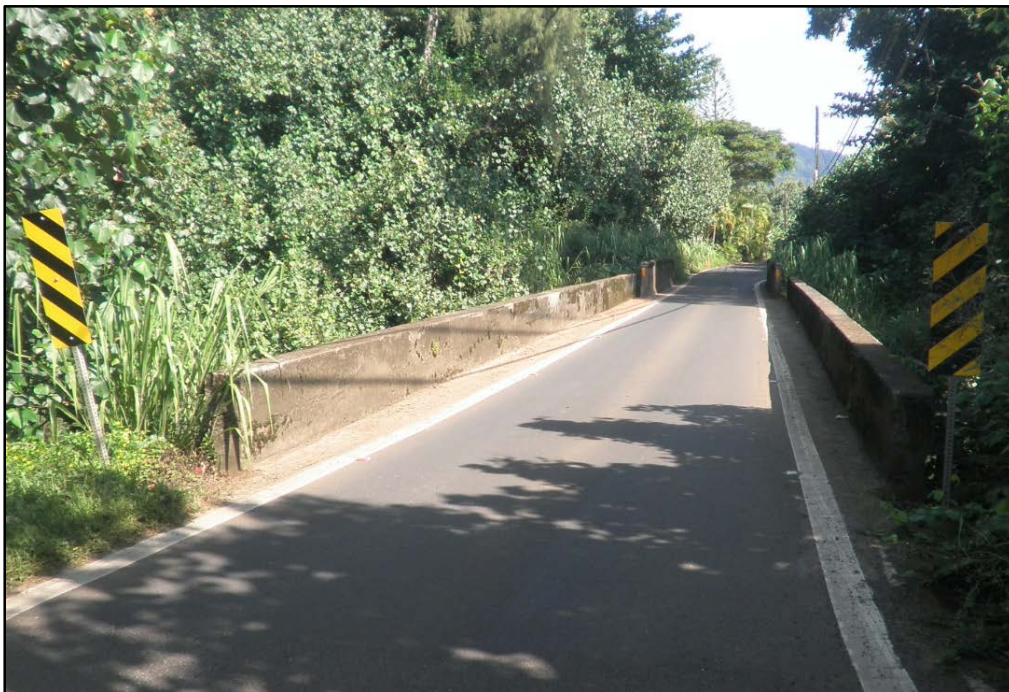
Figure 52. SIHP # 50-30-03-2297, the Waipā Stream Bridge, view to southeast; note the 1925-built concrete bridge extension in the foreground
