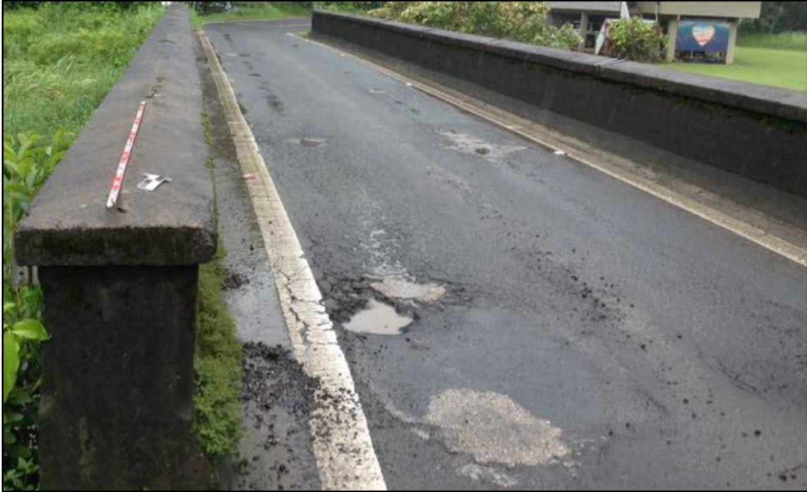
Figure 47. SIHP # 50-30-03-2296, the Wai'ole Stream Bridge, profile view to north
