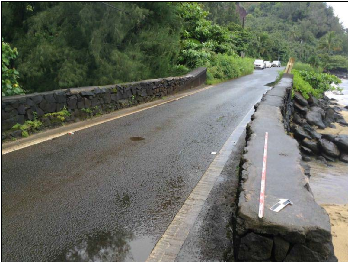
Figure 63. SIHP # 50-30-03-2298, the Waikoko Stream Bridge, general view to northwest
