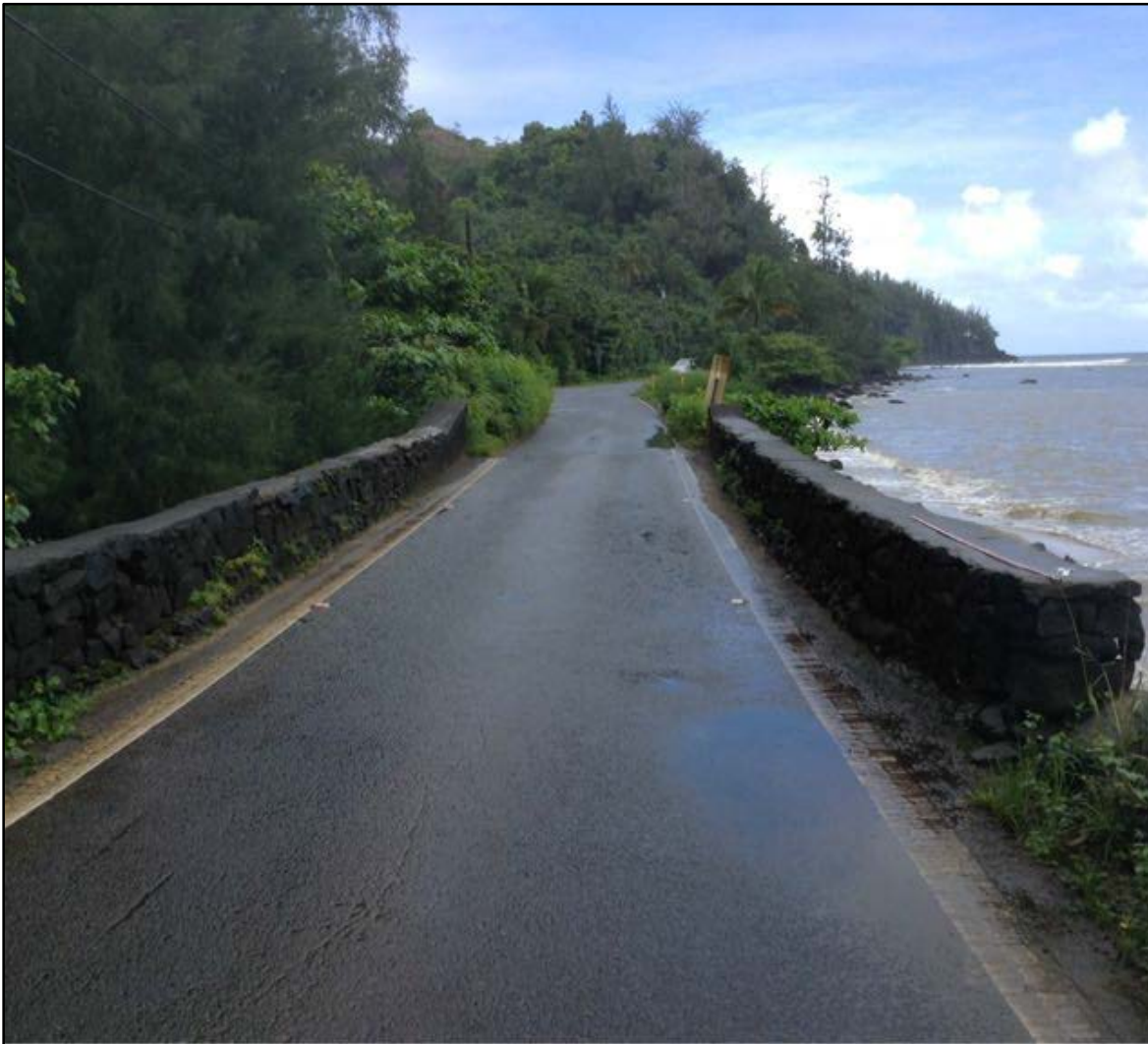
Figure 57. SIHP # 50-30-03-2298, the Waikoko Stream Bridge, general view to north
