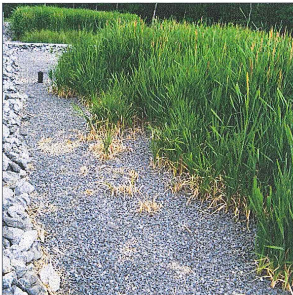
Figure 3: Image of a Subsurface Flow Constructed Wetland
