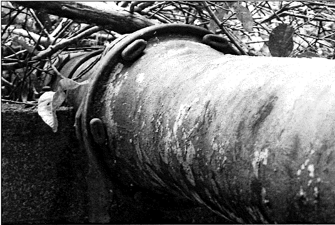
Figure 13. Eight-inch diameter cast iron steel pipe in Gulch 3.
