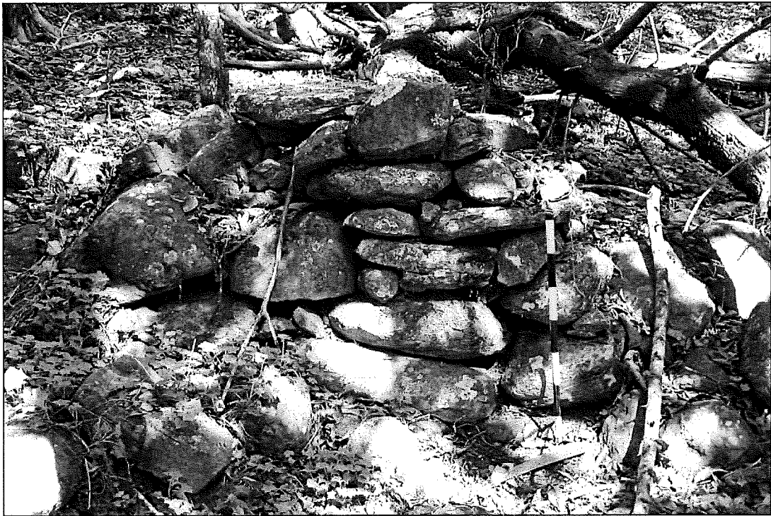
Figure 10. Close-up of modified retaining wall.
