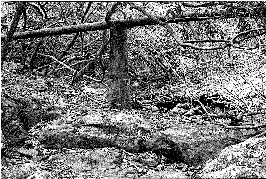
Figure 14. Eight-inch diameter steel pipeline extending across the floor of the gulch.
