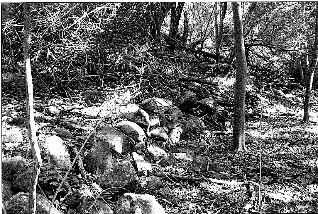
Figure 7. Site 50-50-06-6273, slope retaining wall and soil terrace. View to north.
