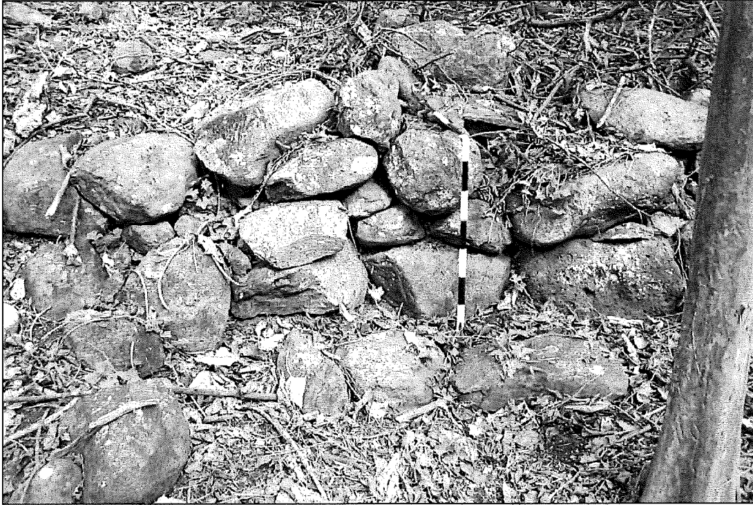
Figure 9. Close-up of retaining wall. View to west.
