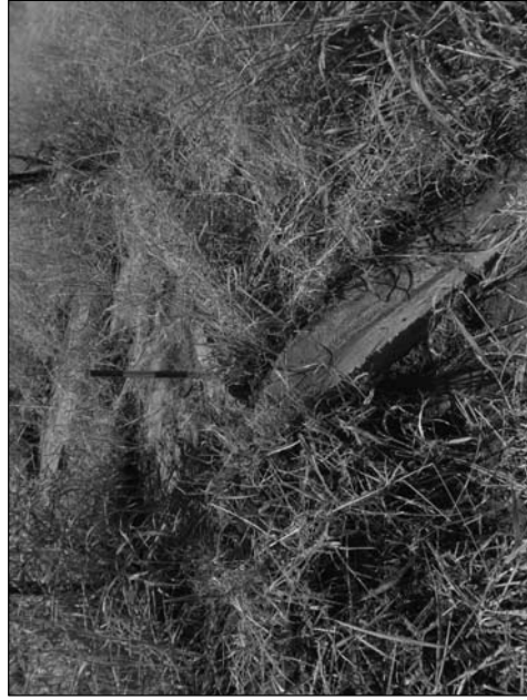
Figure 71. Site 2570, concrete drainage trough (view south).
