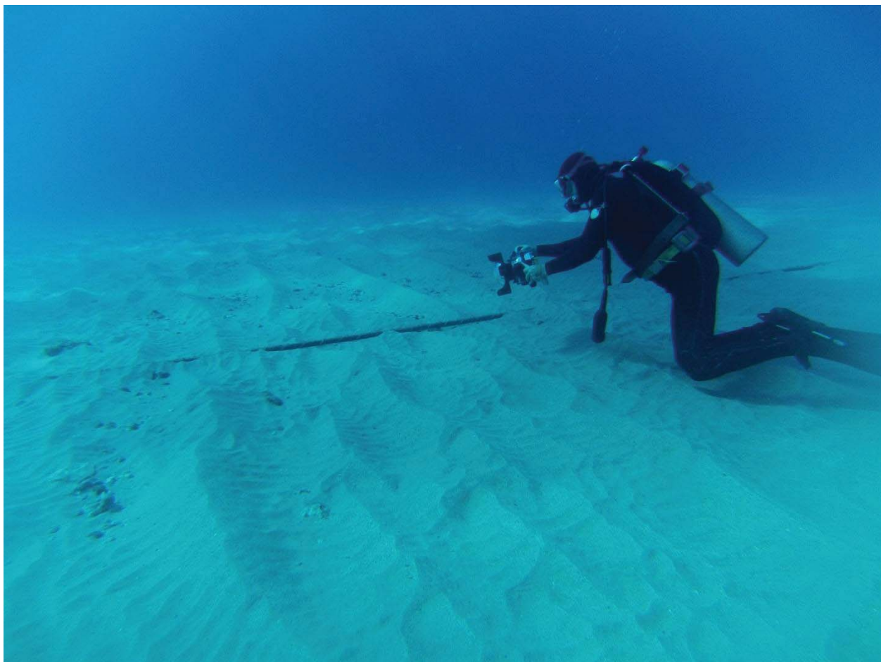
Figure 5. Exposed existing cable
