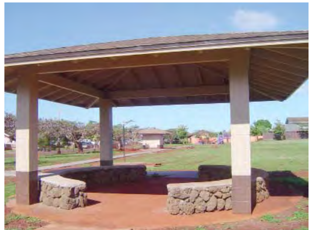
Pavilion at Hanapēpē Cliffside Park
