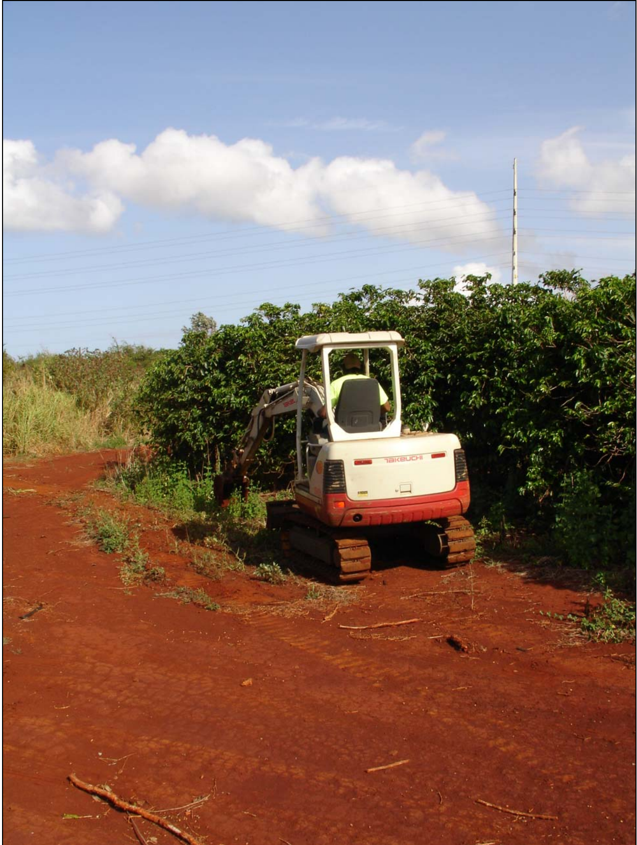
Figure 16: Photograph showing Location of Trench #3, Pre-Excavation. View to North.
