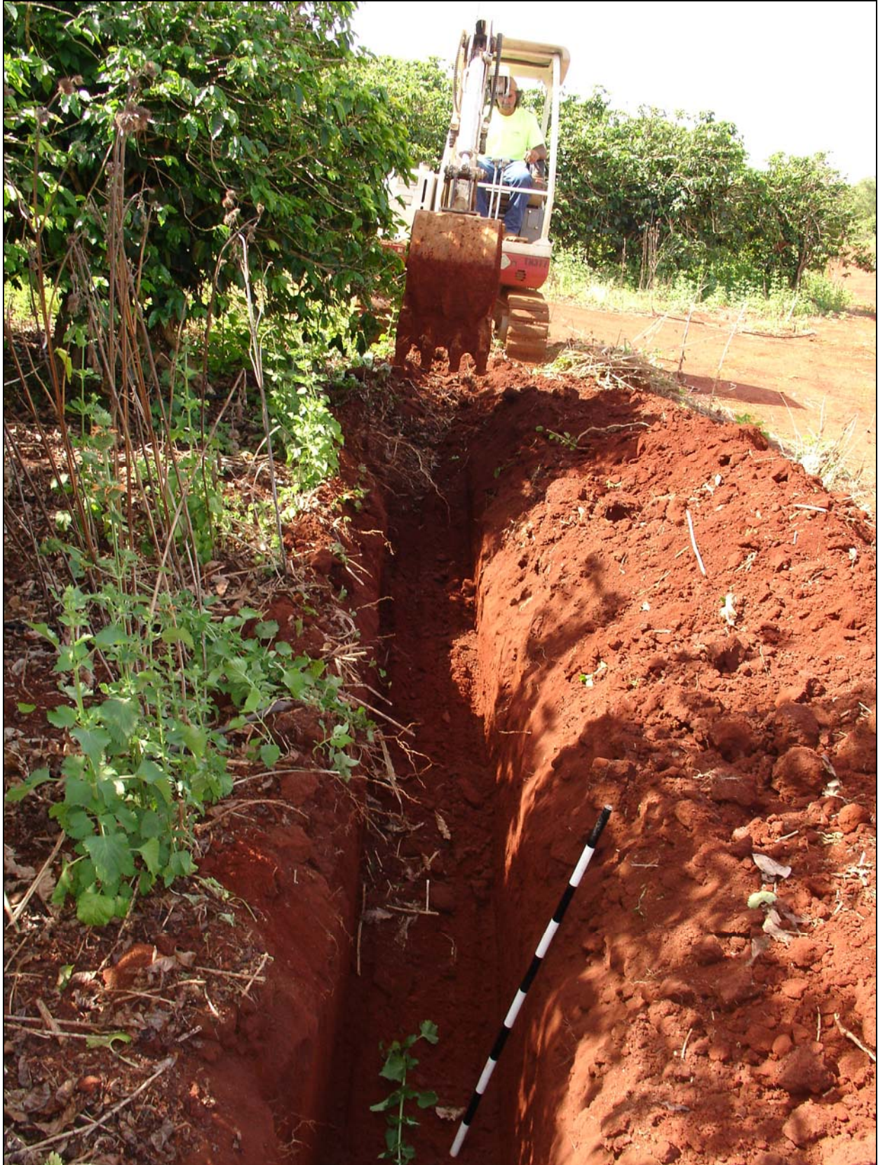
Figure 15: Photograph of Trench #4 Stratigraphy. View to West.
