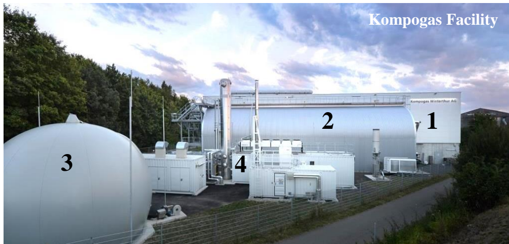
Figure 3-1 Example of a plug-flow anaerobic digester facility: (1) material receiving building; (2) horizontal plug-flow digester; (3) biogas storage tank; (4) biogas upgrade system
