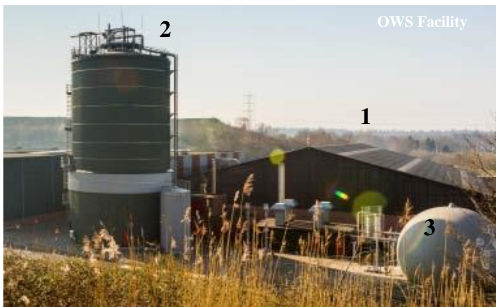
Figure 3-2 Example of a high-solids anaerobic digester facility: (1) material receiving building; (2) vertical plug-flow digester; (3) biogas storage tank
