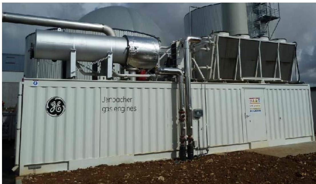
Figure 3-9: Example: CHP unit in Container with heat Recovery and Cooling System
