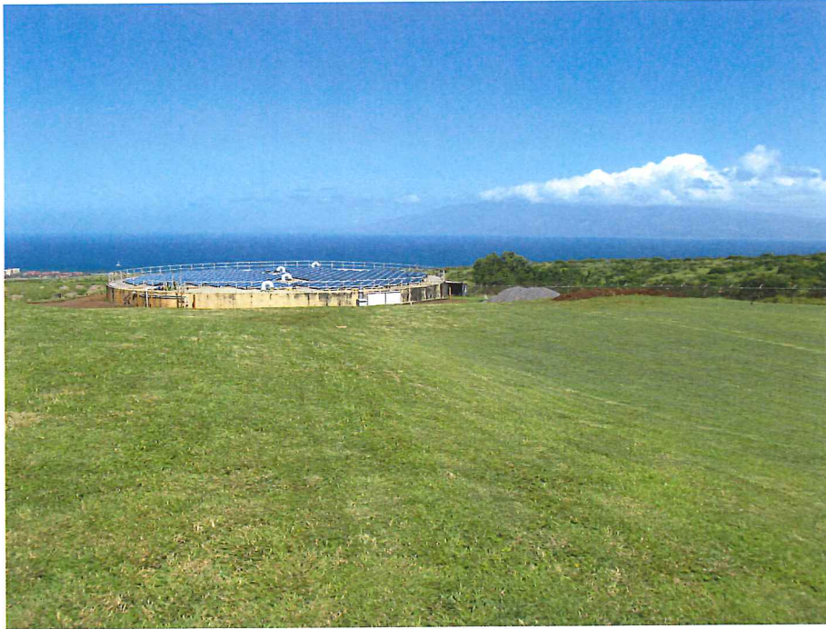
Photo No. 1: Northwest view toward project site
