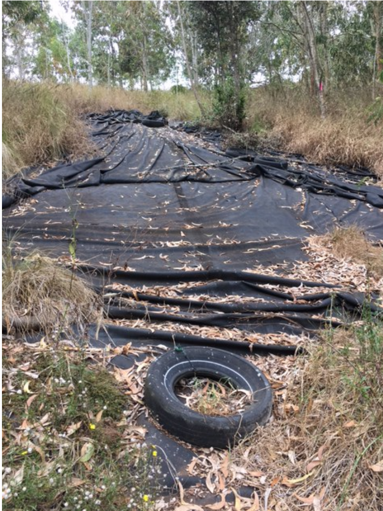
Picture 2: Lower Poohohoo reservoir looking at the south-side of the embankment (facing north). Visible is the degraded butyl liner, held down by old tires. Plants are growing out of the liner including fountain grass, fireweed, molasses grass, 'ōhi'a, and koa all visible in this picture.
