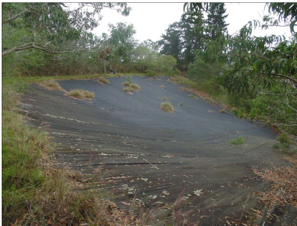
Figure 21. Butyl-rubber lining on interior slopes of reservoir area, view to southeast
