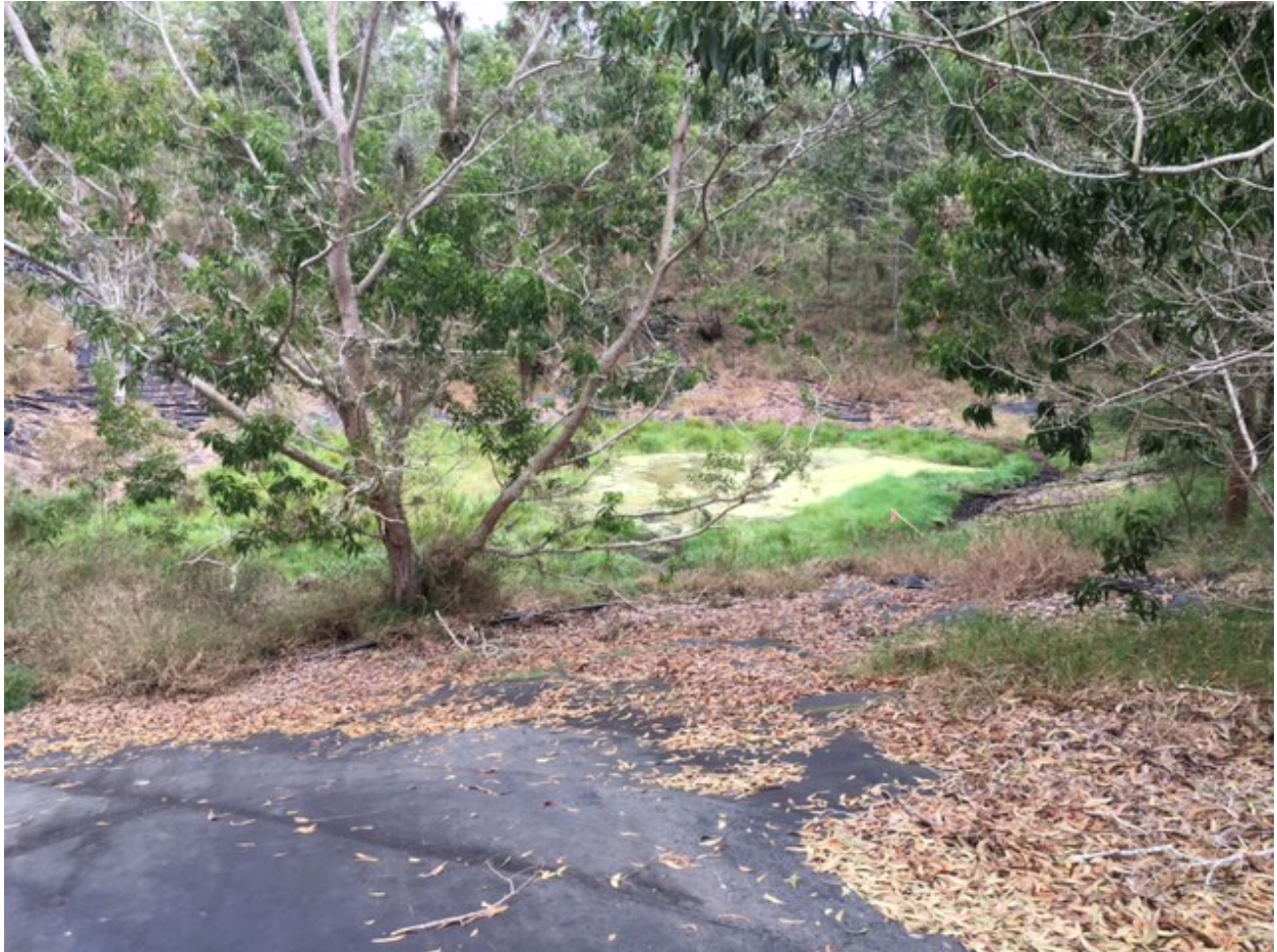
Picture 3: View looking north into the bottom of the reservoir where large koa have grown out of holes in the butyl liner. The very bottom of the reservoir contains water and vegetation, and likely plenty of mosquito larvae. Only non-native birds were observed to drink and bathe in the water.
