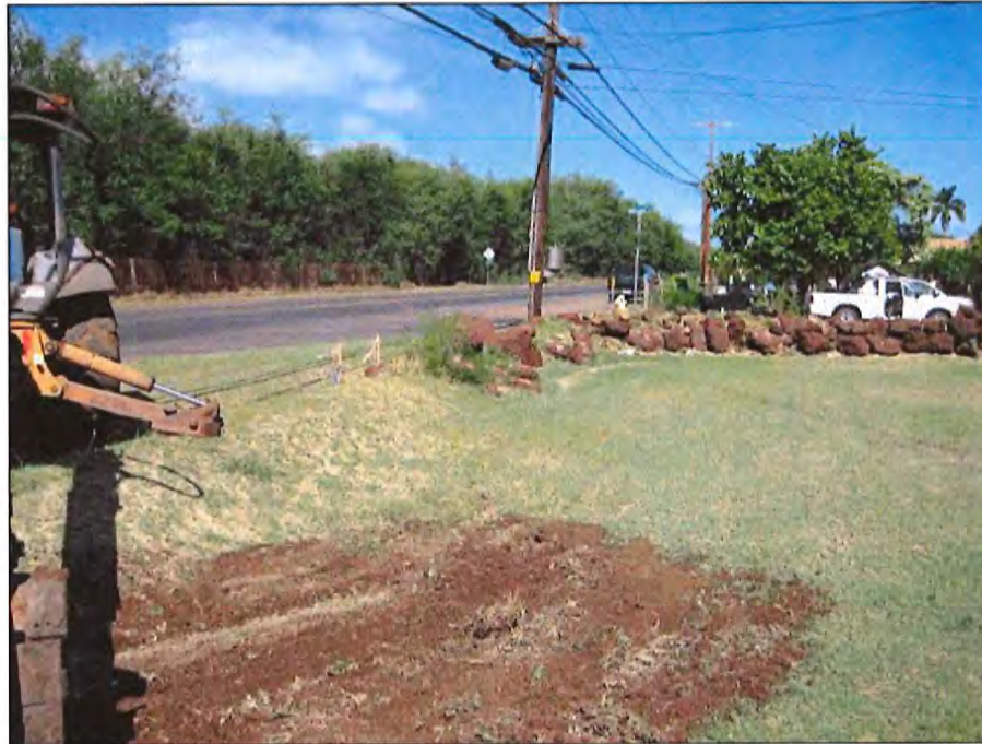
Figure 15. Section of restacked wall along Kapa'akea Loop Road, facing east.
