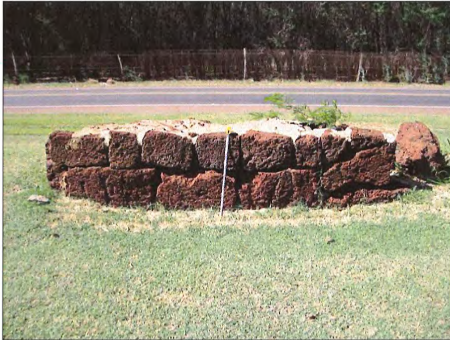
Figure 13. Rock and concrete wall, facing north.
