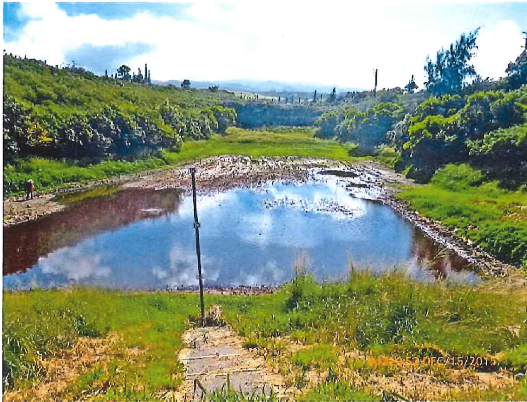
Figure 4. Desilting basin in Nāpili 4-5 located upstream of project area.
