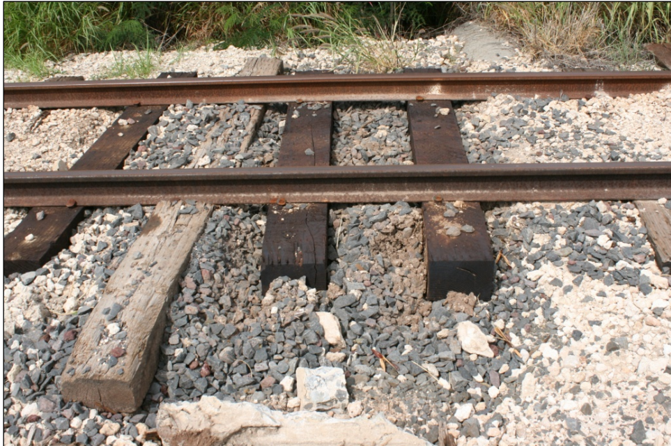
Figure 9. Close-up view of repaired track at Site 50-80-12-9714, showing new ties and gravel.
