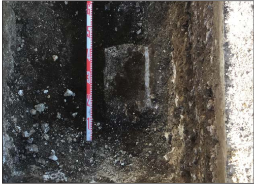
Figure 101. Photograph of SIHP # -7942, Feature 2d concrete blocks in southeast corner of T-3; plan view
