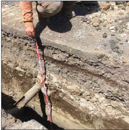
Figure 44. Photograph of utility pipe in T-3 Stratum Ie
