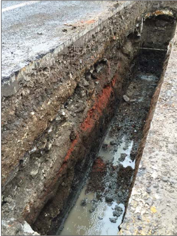
Figure 29. Photograph of T-1 at base of excavation; view to northeast
