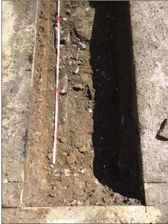
Figure 96. Plan view photograph showing SIHP # -7942, Feature 2a concrete block alignment exposed at 60 cms in southwest half of T-1
