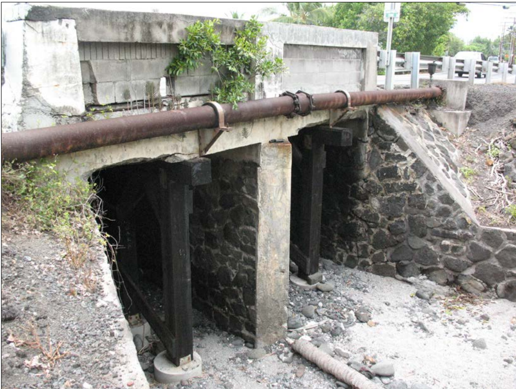
Figure 7. Recently installed wooden post and beam support structure below bridge, view to the northwest.
