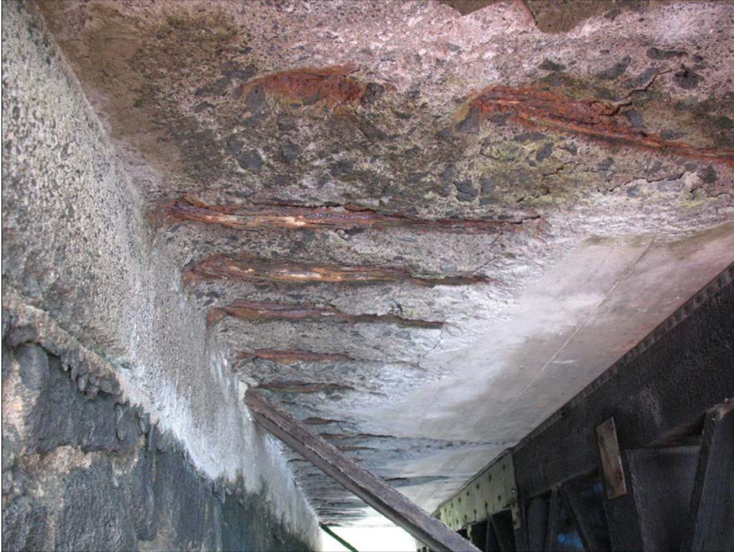
Figure 6. Detail of underside of Kahului Bridge deck showing concrete spalls with exposed iron.
