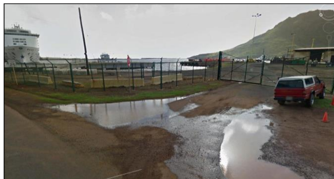
Photo 2-1. Poned Storm Water at Wa‘apa Road and Harbor Access Road Gate Photo Credit: Google Earth, Accessed March 19, 2017
