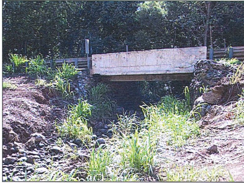
Figure 3. Honolua Stream Bridge view E from streambed.
