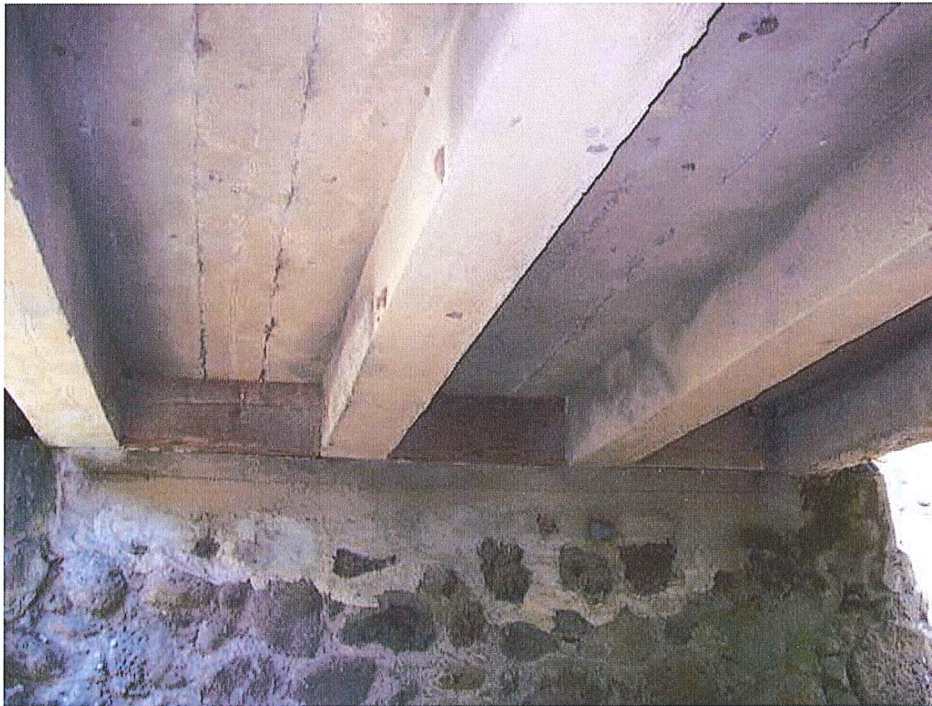
Photo 4 – Underside of bridge
