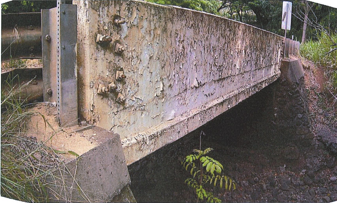
Photograph 7. HI_MauiCounty_HonoluaStreamBridge_0007. Outboard side of the upstream parapet. Note the beveled string course at the lower edge of the parapet. View facing northwest.
