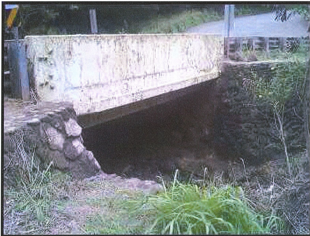
Figure 14: View South of SIHP No. -1754 Showing Bridge
