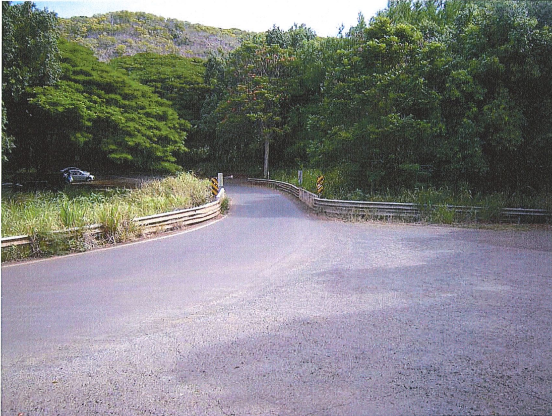
Photograph 3. HI_MauiCounty_HonoluaStreamBridge_0003. Wide overview of the bridge showing the rural setting with a parking area in the left background. View facing north.
