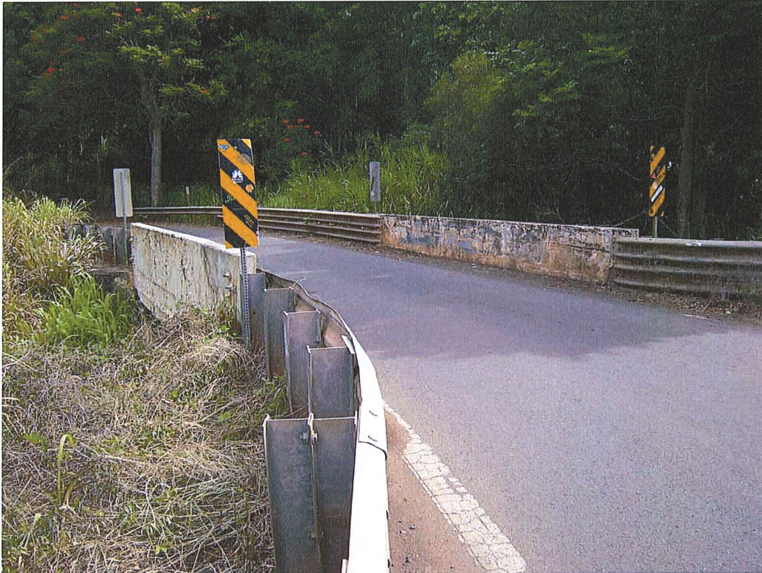
Photograph 2. HI_MauiCounty_HonoluaStreamBridge_0002. Overview of the bridge showing the plain, solid parapets. View facing northeast.
