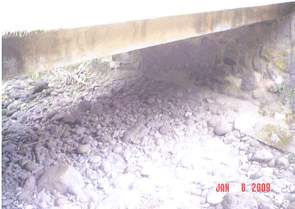
Photo 2 – Streambed under bridge structure
