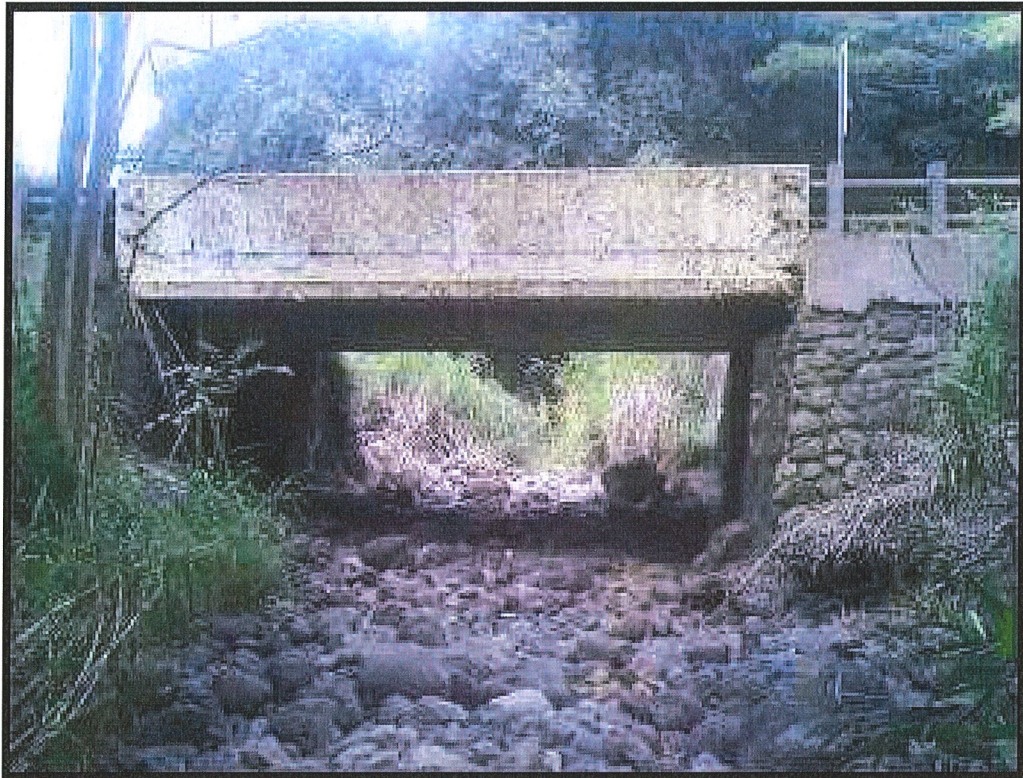
Figure 13: View East of SIHP No. -1754 Feature 11 Showing Bridge Crossing Honolua Stream
