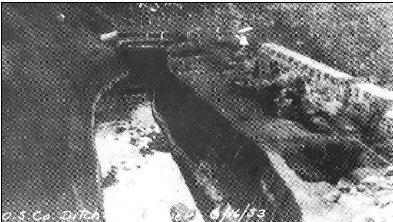
Figure 20. Oahu Sugar Company irrigation ditch under construction in 1933 at Kīpapa Gulch (Bishop Museum)
