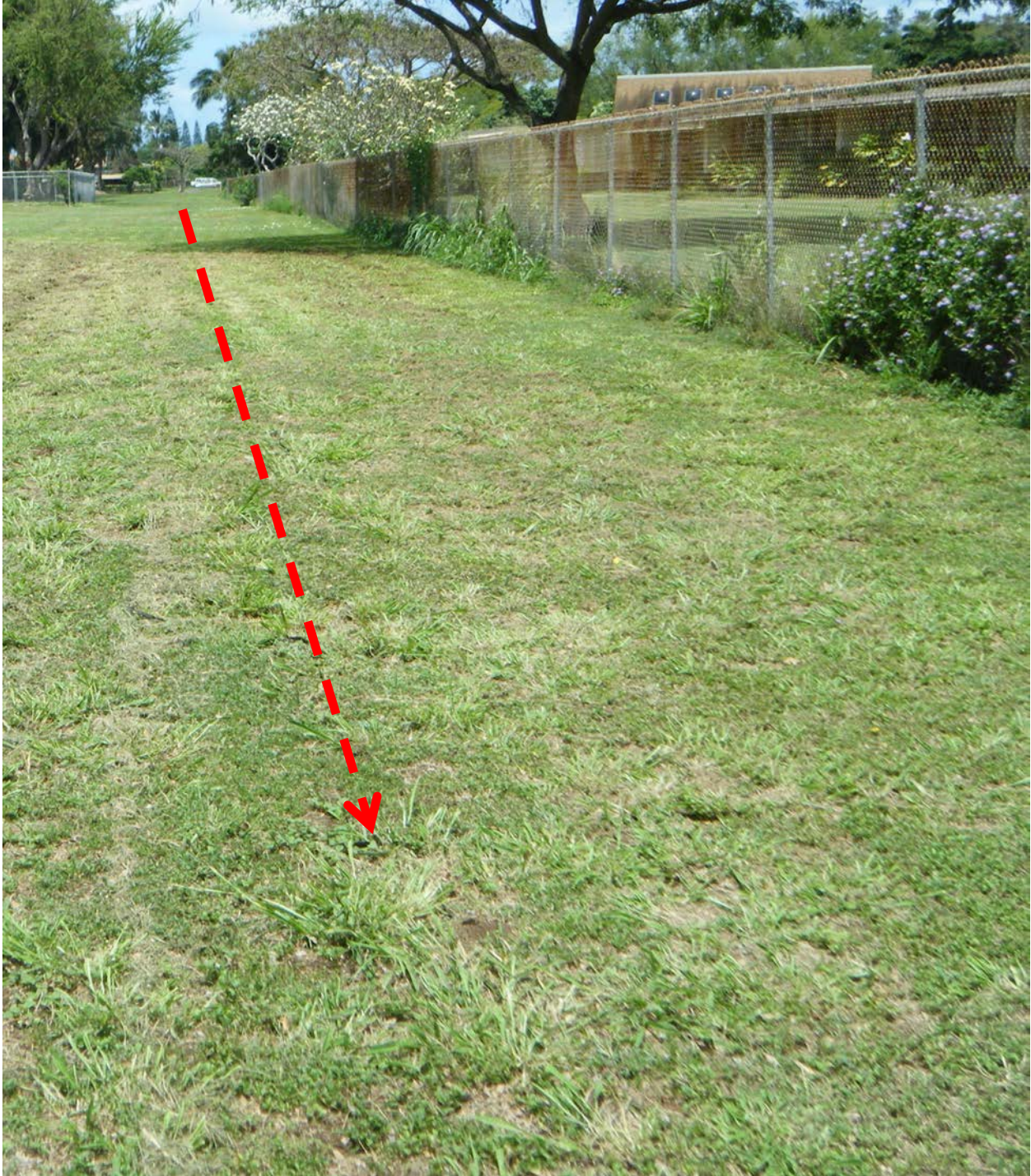
Figure 3B. Drain alignment. Underground drainage system alignment adjacent to Haleiwa Elementary School Fence. The drain inlet would be in the far background of photo. Direction of water flow (red arrow) would be from the far background to the foreground where the drain would exit to Kaiaka Bay.
