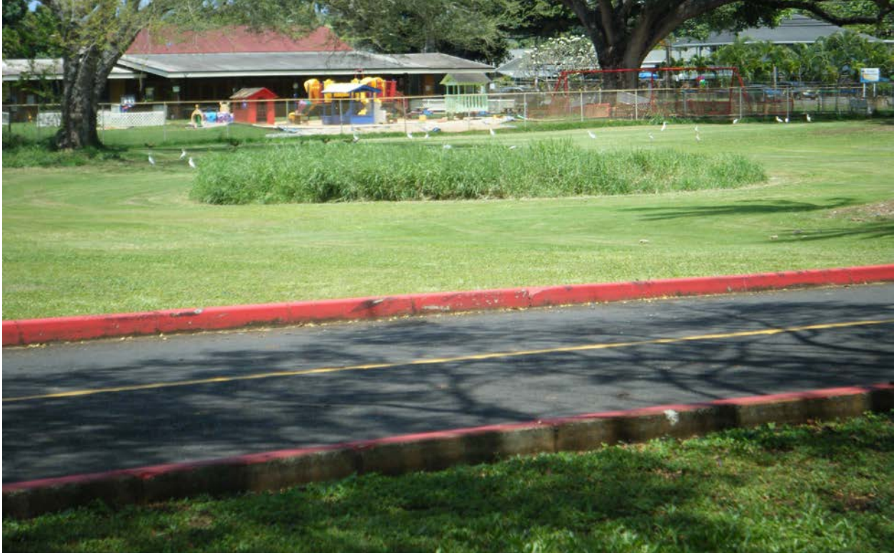
Figure 3A. Depression in Park. High grass grows in the center of the depression in the park where water ponds. In the background is the First Baptist Church Preschool. Foreground is the Kaiaka Bay Beach Park interior road. The drainage system will pass beneath this road.
